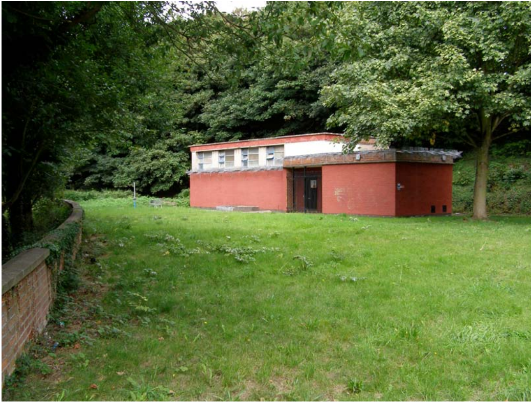
Plate 13: Spital Dam Sewage Pumping Station, 22/08/2006
