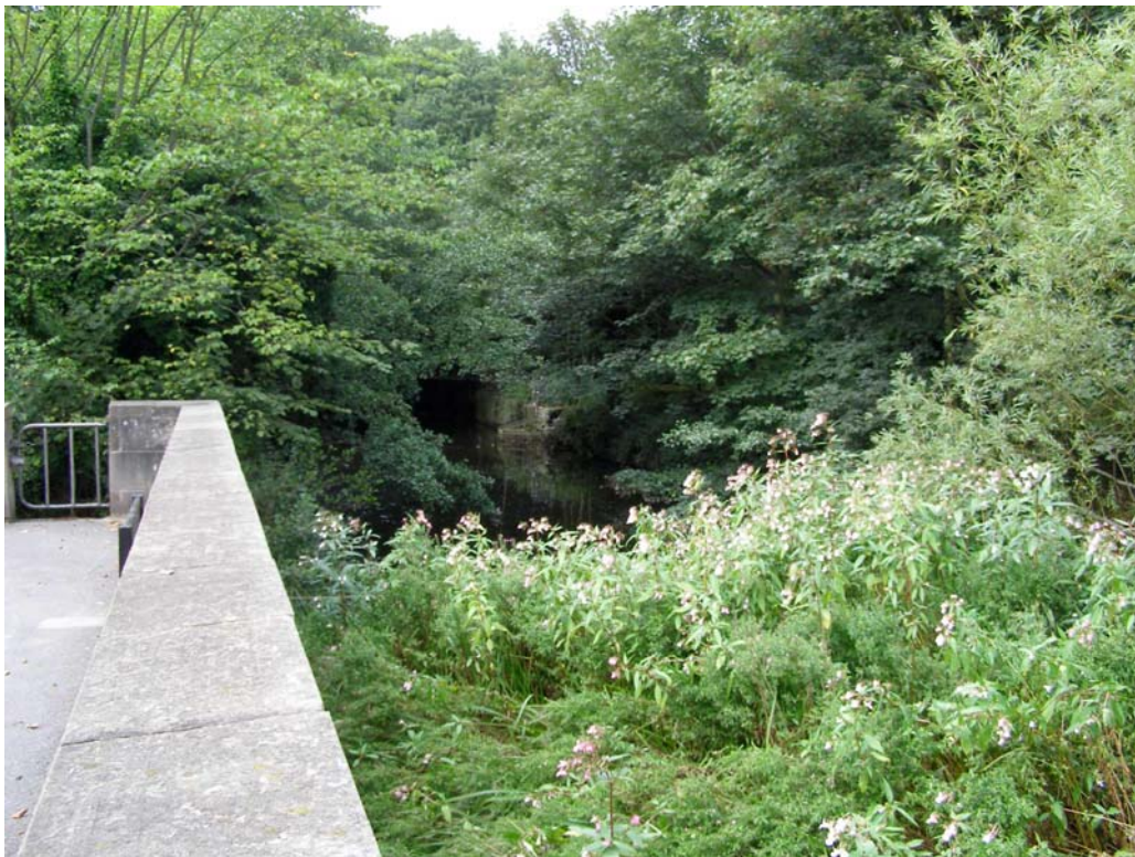
Plate 12: View north-north-east from Spital Dam, 22/08/2006
