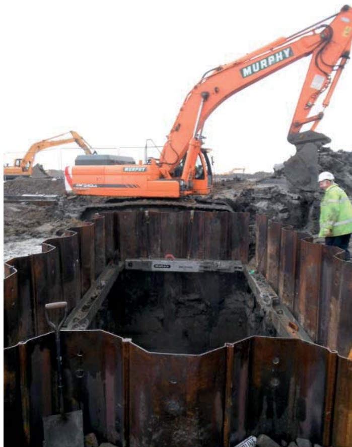
Plate 10: Deep drainage excavations in progress
