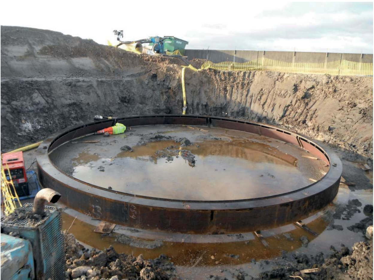
Plate 8: Plate 8: Deep drainage excavations in progress (pumping station)
