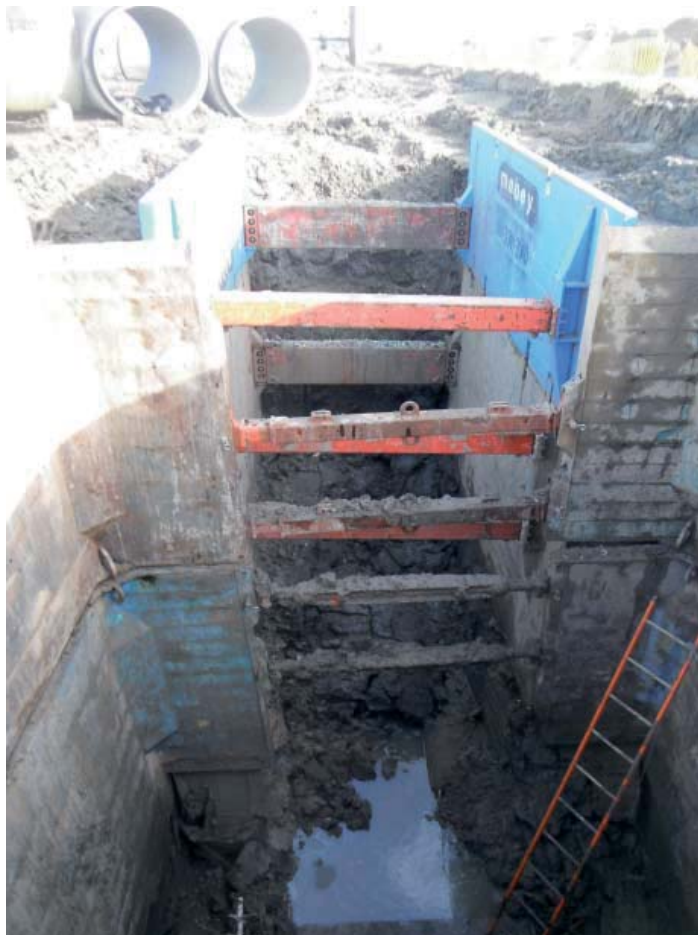
Plate 4: Deep drainage excavations in progress
