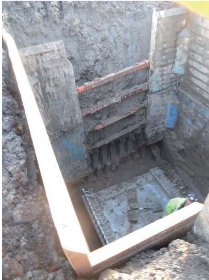
Plate 3: Deep drainage excavations in progress
