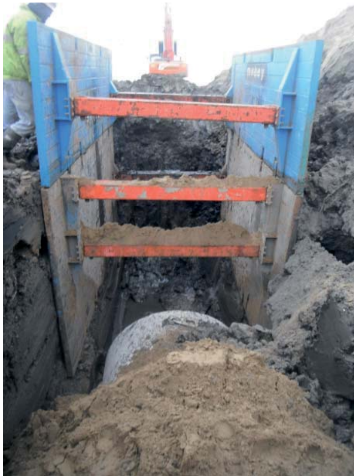
Plate 1: Deep drainage excavations in progress
