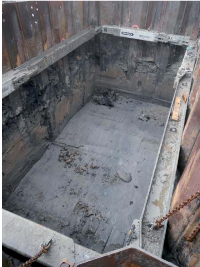
Plate 9: Deep drainage excavations in progress
