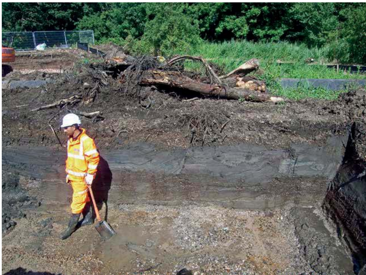
Plate 4: Shallow sequence of alluvium overlying terrace gravel on east side of Mucking Creek valley
