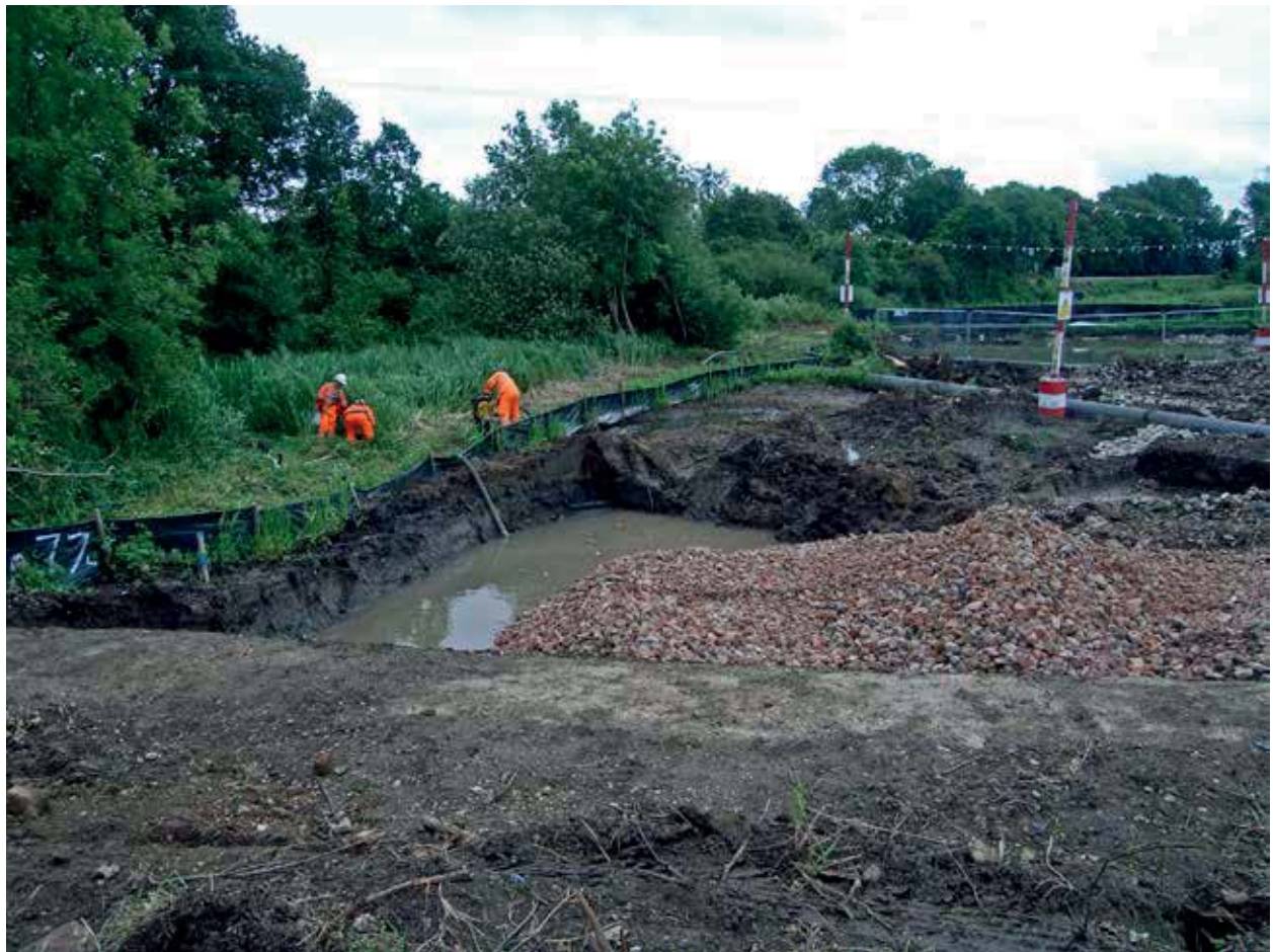
Plate1: Installing piling mats in Mucking Creek
