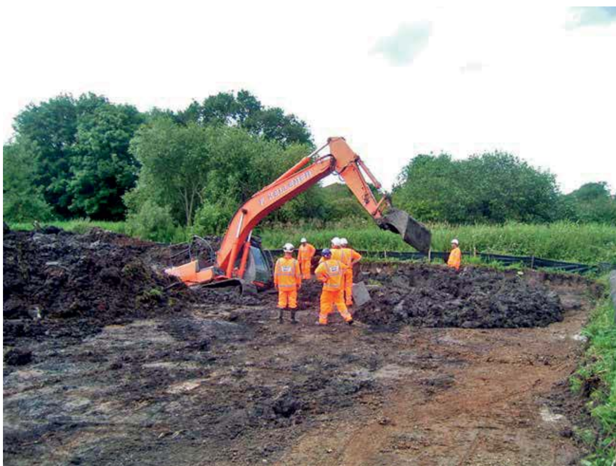
Plate 8: An excavator sinks into the soft, deep peat deposits infilling the valley of Mucking Creek. The surface of the underlying terrace deposits can be seen emerging to the right of the picture, forming the east bank of the stream valley
