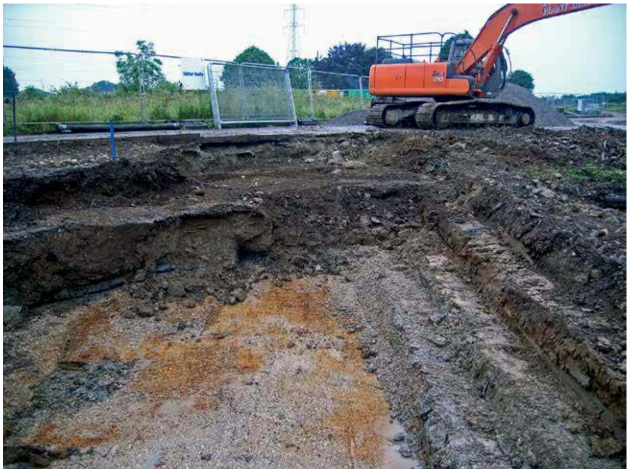
Plate 2: Exposure of terrace gravel beneath made ground on east side of Mucking Creek
