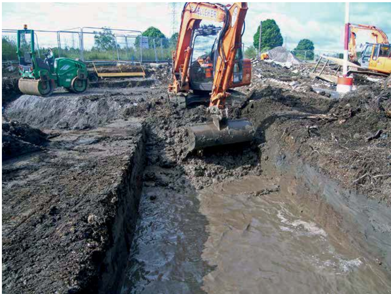
Plate 3: Excavation into upper alluvium adjacent to Mucking Creek
