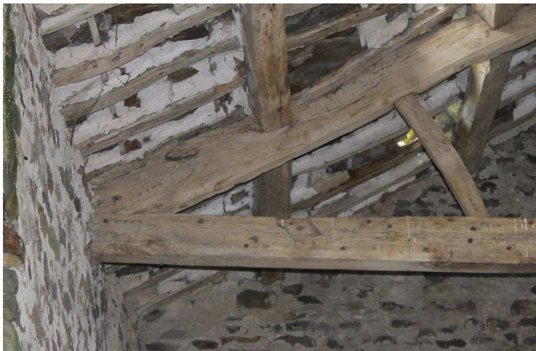
Plate 21: Punched assembly numbers, indicating truss four
