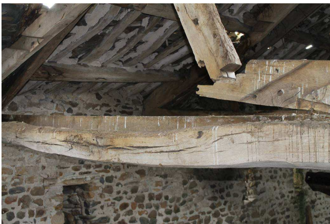
Plate 19: A failed principal rafter on the northern truss. The empty halfting joints can be seen on both rafters indicative of their reuse
