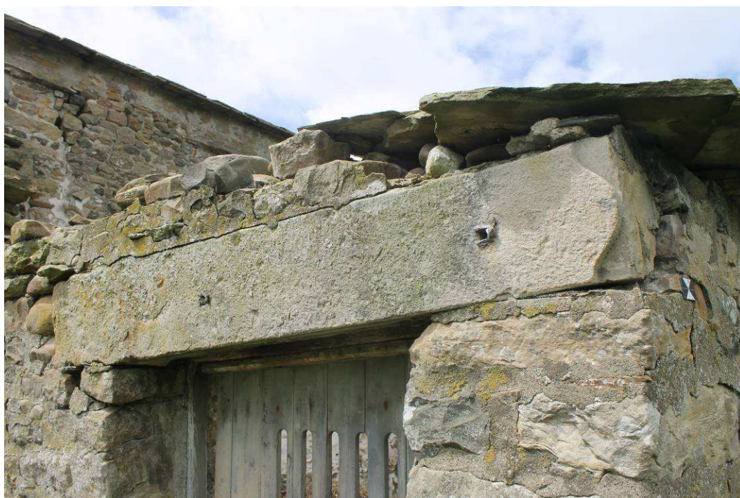
Plate 30: Sandstone gate-post reused as a lintel above the entrance into the south-eastern lean-to
