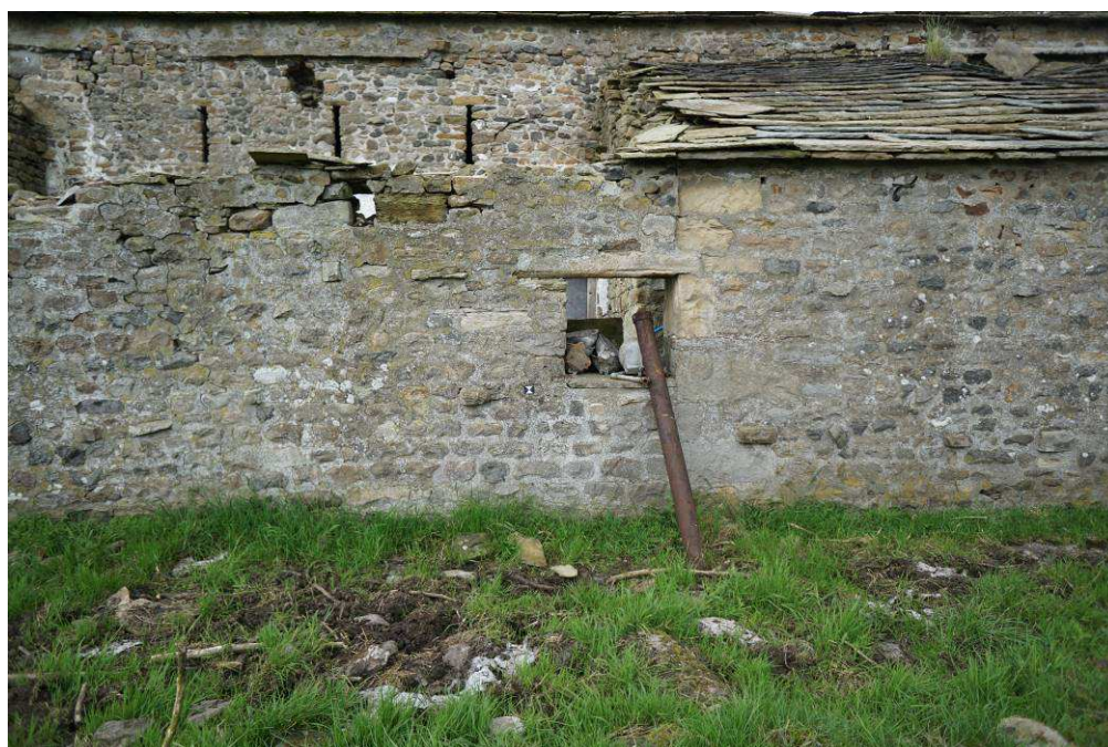
Plate 24: Stone quoins indicating the butt joint between the eastern walls of the north-eastern and south-eastern lean-to, facing west
