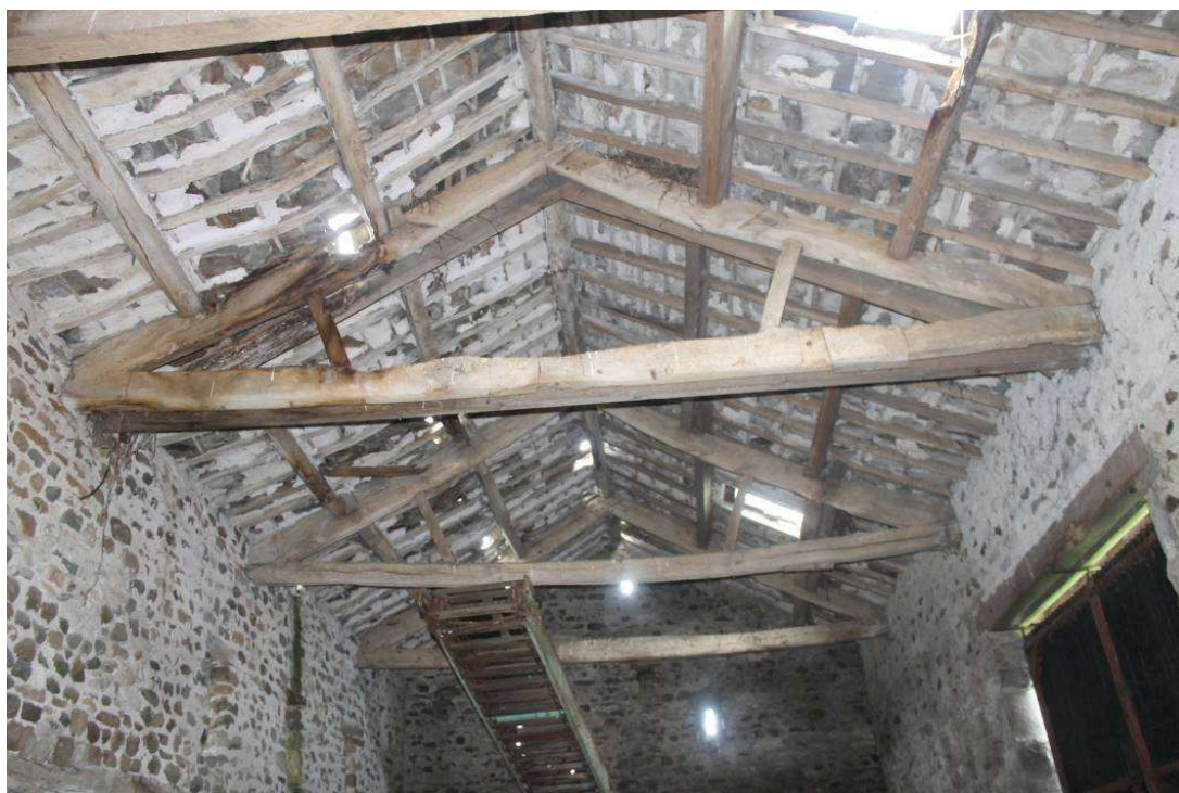
Plate 18: The truss design in the Main Barn
