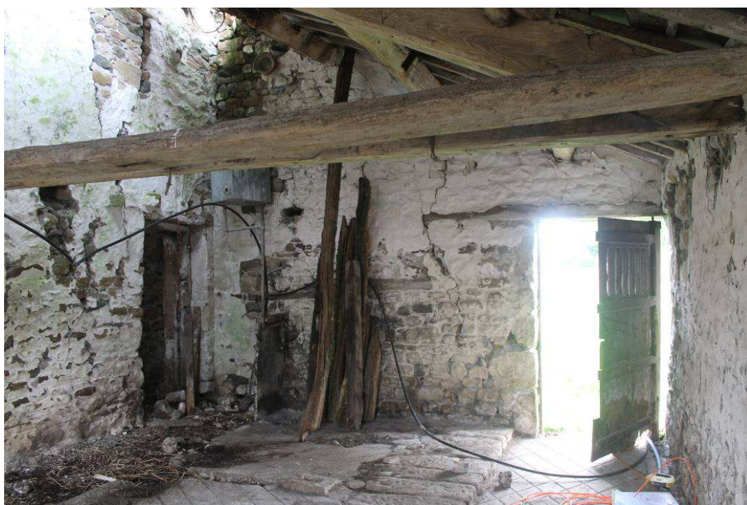
Plate 27: Interior of the north-eastern lean-to facing north. Note the upstanding slate division to the left of frame
