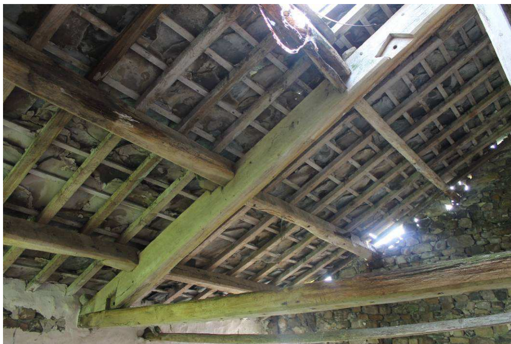
Plate 28: Half truss in the north-eastern lean-to. Note the empty half-timings on the principal rafter, indicative of its original use as a tie beam. Facing south
