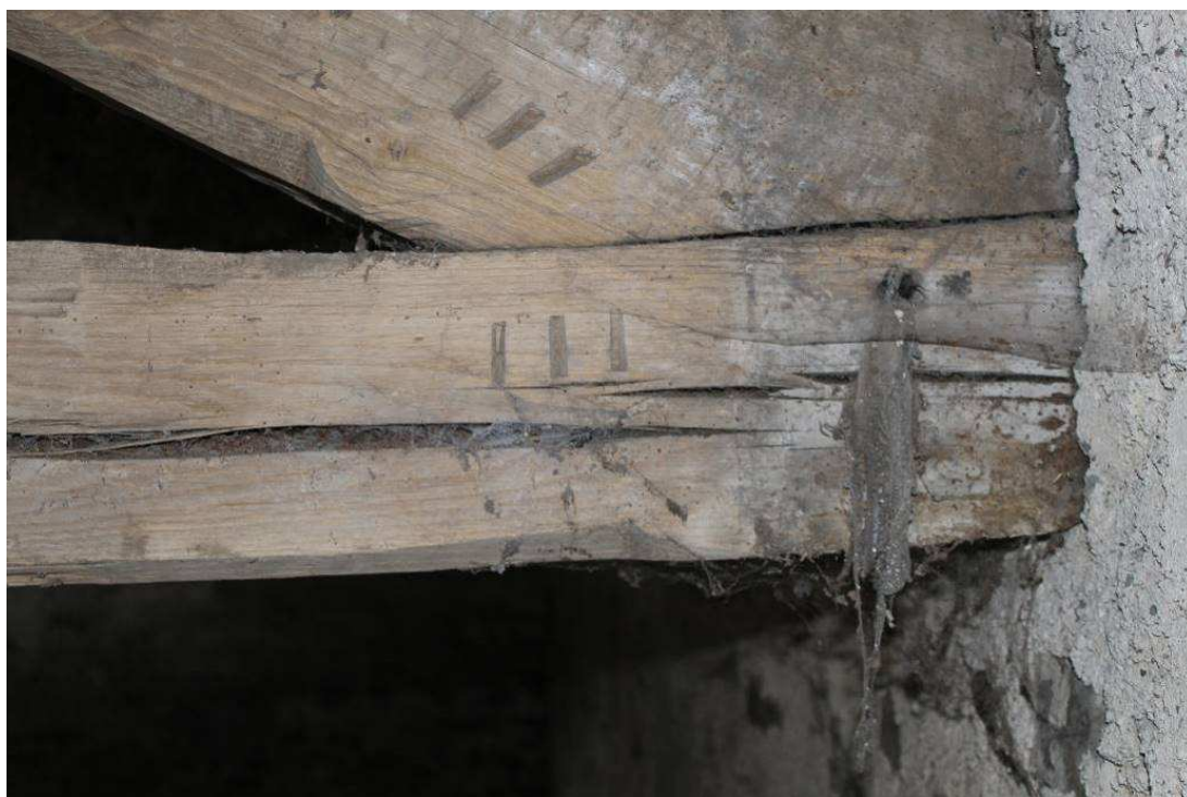
Plate 20: Roman numerals marking assembly order. Note also the chamfered stops on the underside of both beams
