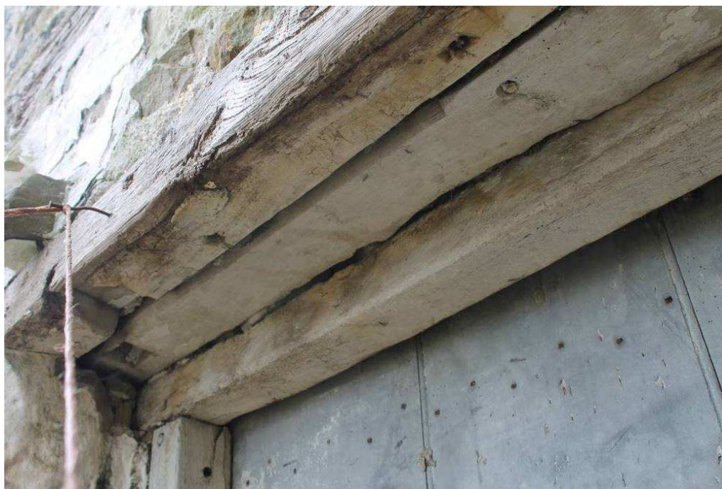
Plate 12: Underside of the lintel of the central eastern door showing reused timbers
