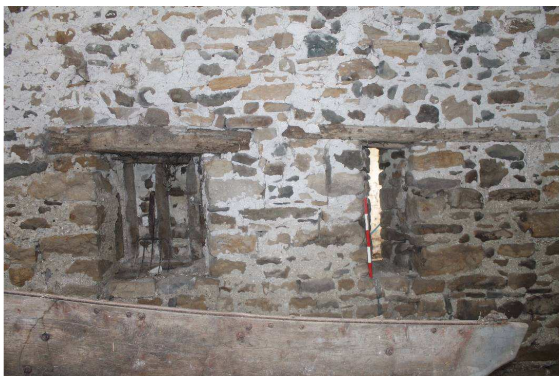
Plate 17: Blocked window and vent at the northern end of the eastern elevation
