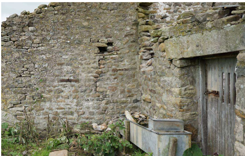
Plate 35: Area of disturbed masonry at the northern end of the eastern wall
