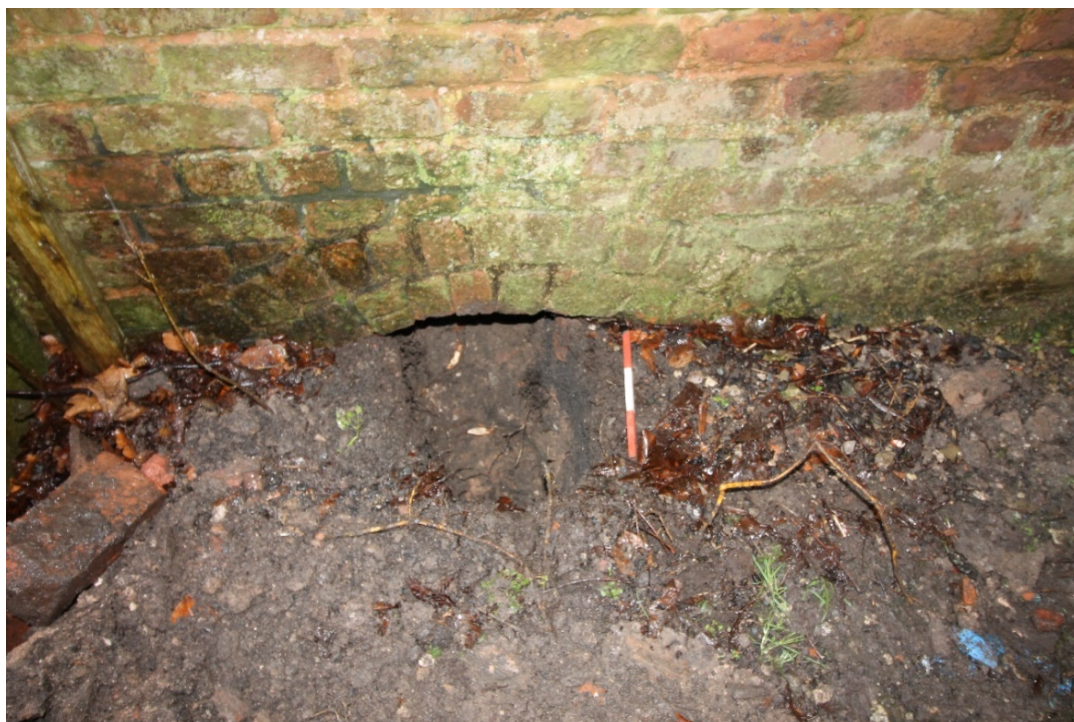
Plate 27: TP 8 excavated in the vicinity of an apparent sub-surface arched opening beneath an ancillary building west of the Stables
