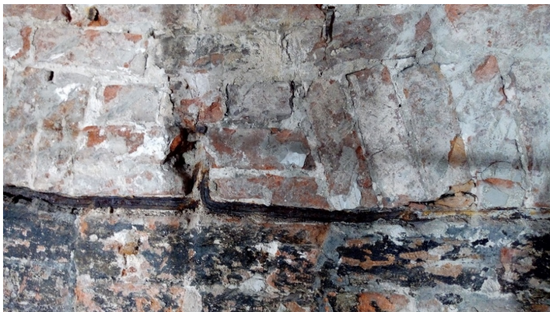
Plate 29: Iron straps supporting the brickwork arches
