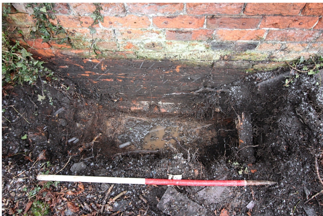
Plate 7: Example of brick footings: TP35 , southern elevation of the Coach House, 1m scale
