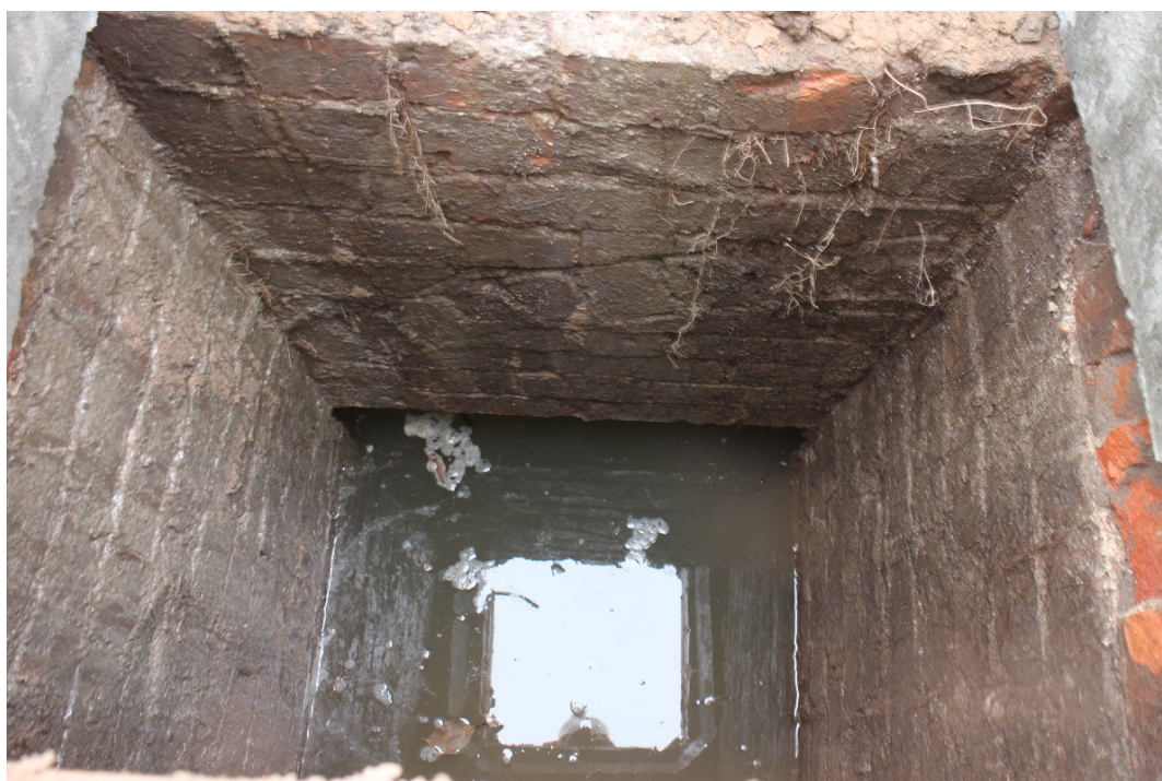
Plate 48: detail of brick-built water tank between the Sunken Garden and south-western extent of the Walled Garden
