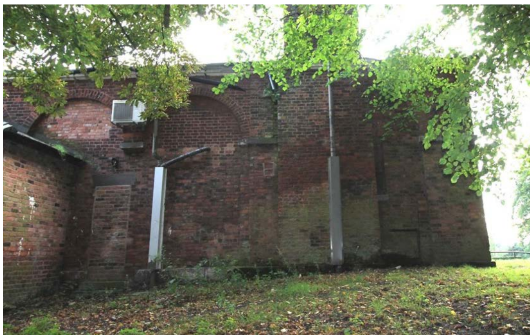
Plate 30: South-western external wall showing chimney stack, blocking window and southern arcade
