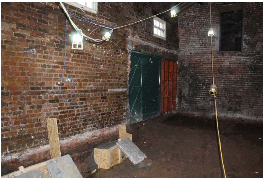
Plate 22: General shot of inside northern wall (B1) of Building B showing wall foundation, present wagon door and rubblestone ramp
