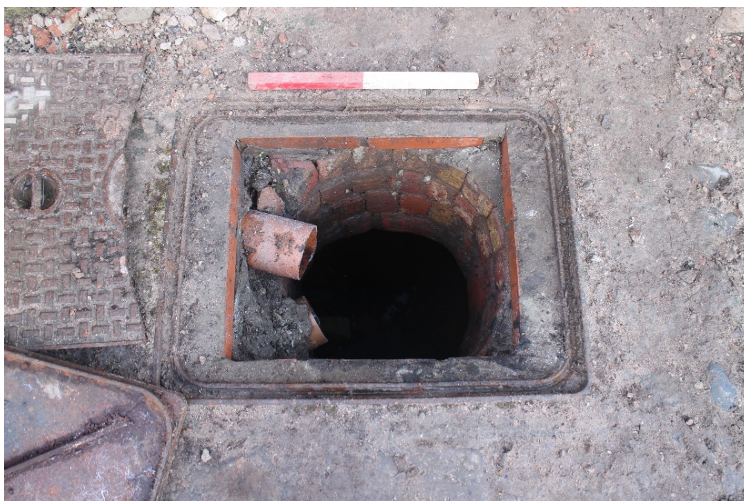
Plate 25: Manhole into the roof of the cistern
