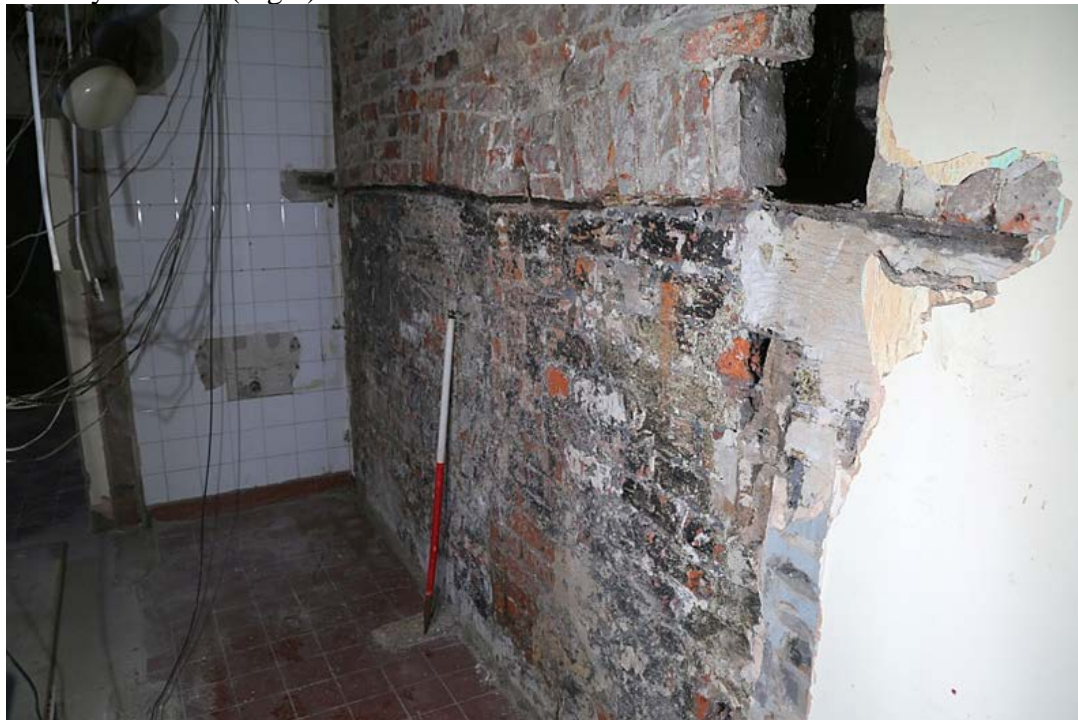
Plate 28: Bricked-up fireplaces with the southern element of the Stables, showing the void behind, 1m scale
