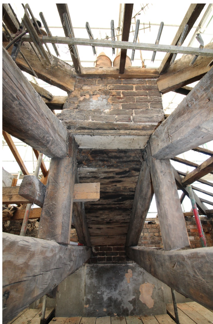
Plate 34: View from the underside of the trusses supporting the lateral stack
