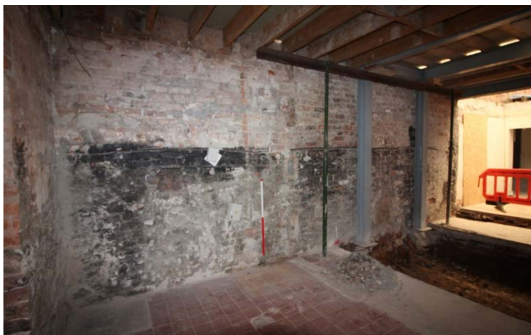
Plate 32: Western wall of the southern element of the Stables, showing the series of arched fireplaces and lift shaft trench
