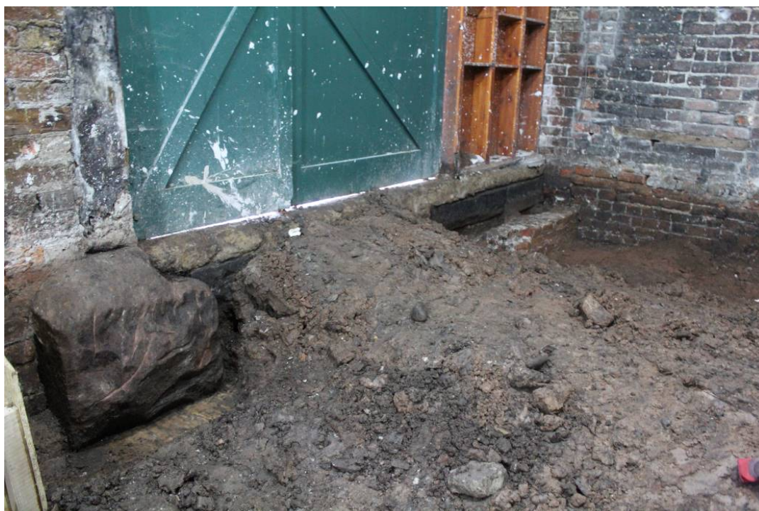
Plate 21: Sandstone plinth, thresholds and wall footings associated with a former wagon door entrance
