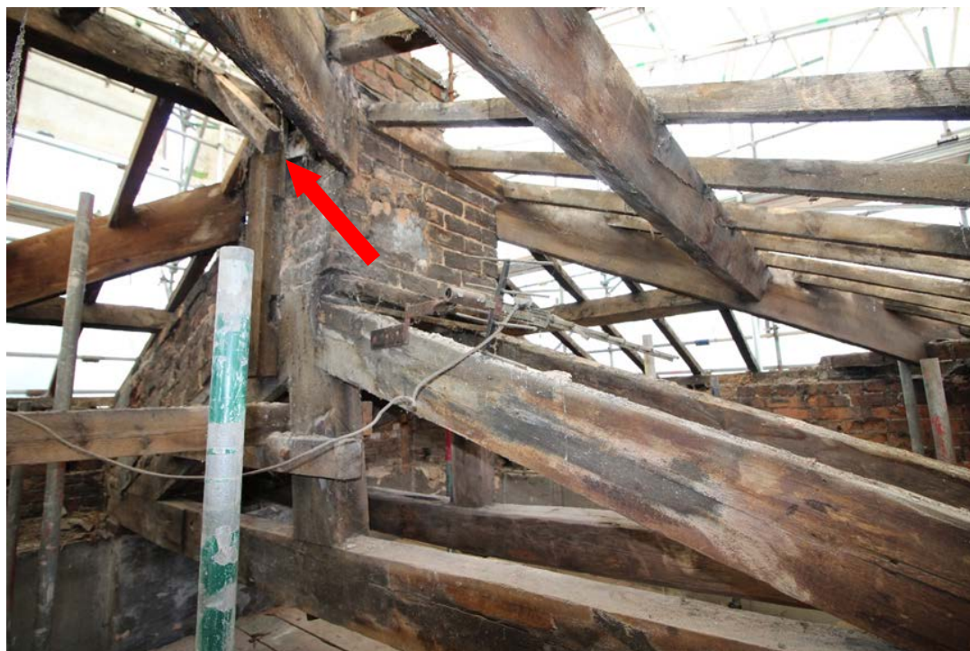
Plate 35: On the south side of the chimney a ridge (marked by an arrow) has been added, superseding the hipped roof structure
