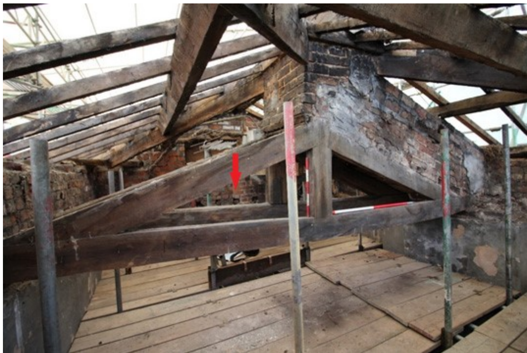
Plate 33: The central chimney, set upon a pair of kingpost trusses, facing south (nb the scaffolding boards do not reflect a former floor level)
