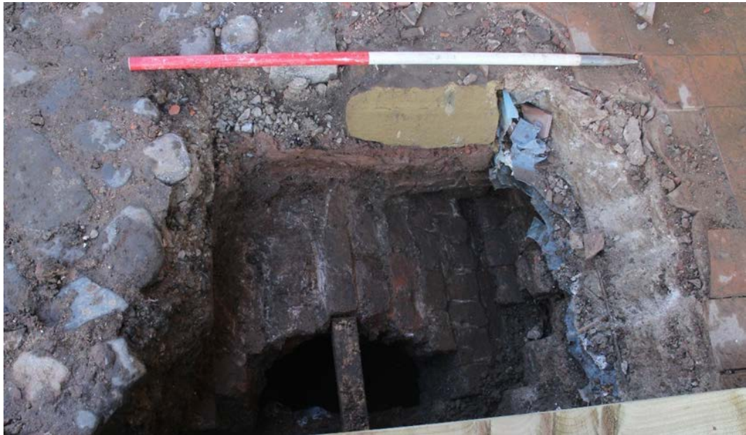
Plate 23: Brick-arched roof of cistern and levelling layers, facing east, 1m scale
