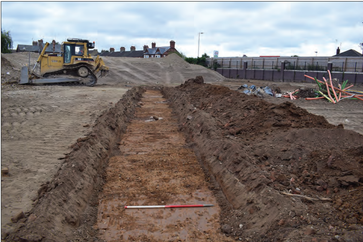
Plate 4: Trench 7, looking north-east
