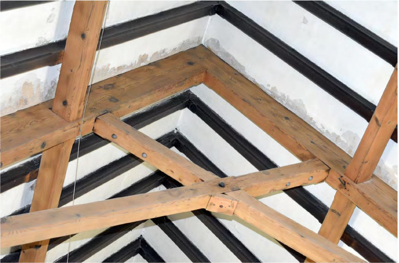
Plate 42: Detail of scissor brace roof
