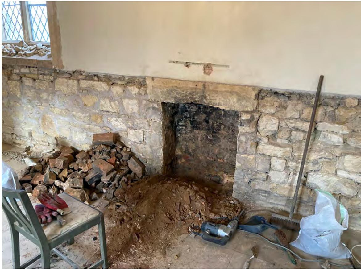
Plate 68: Fireplace in north wall after removal of blocking (photo provided by Geoff Bolam)
