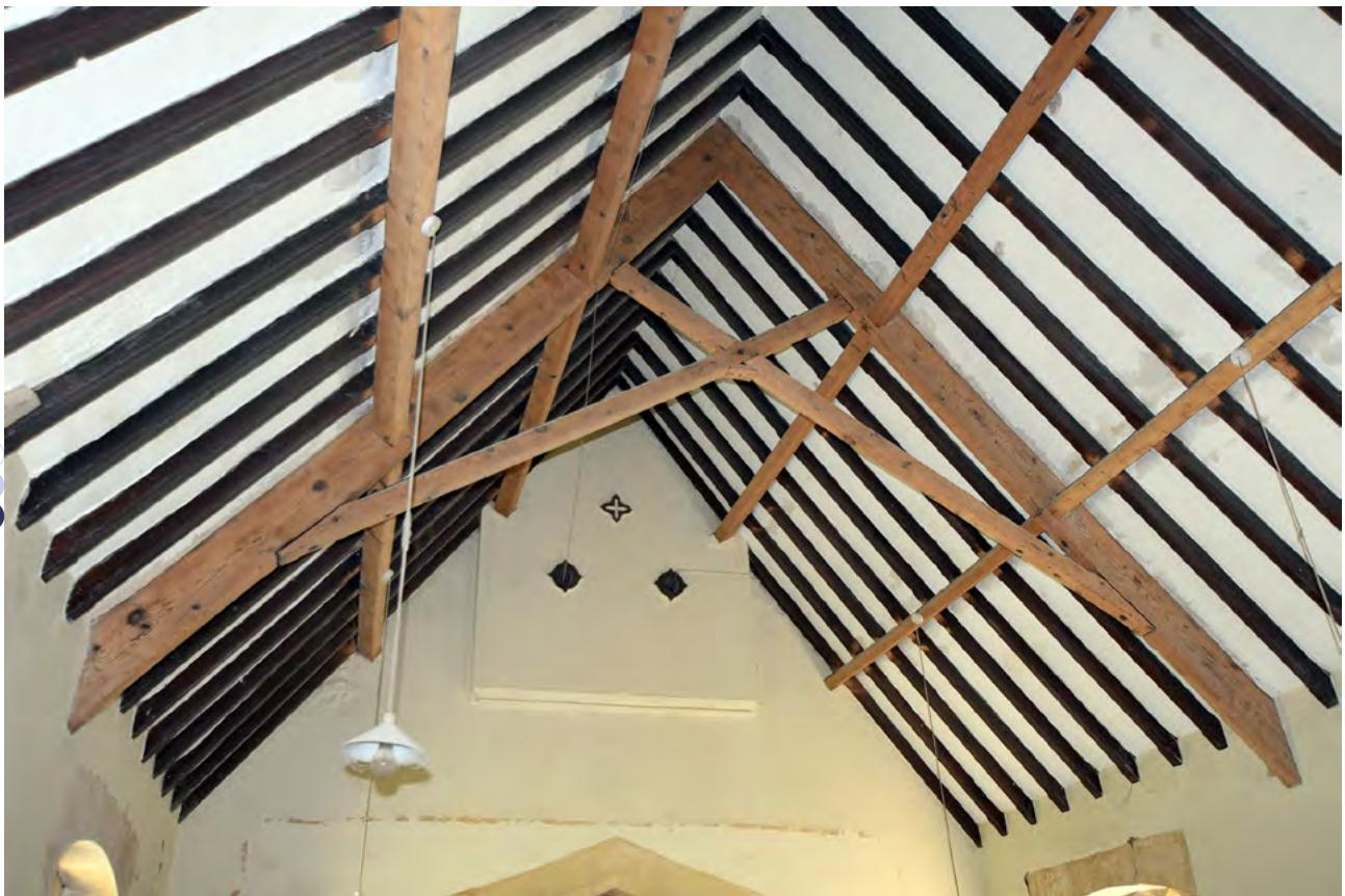
Plate 40: Scissor brace roof looking east
