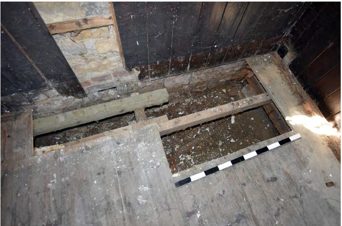
Plate 61: Exposed floor joists at south-west corner of school room
