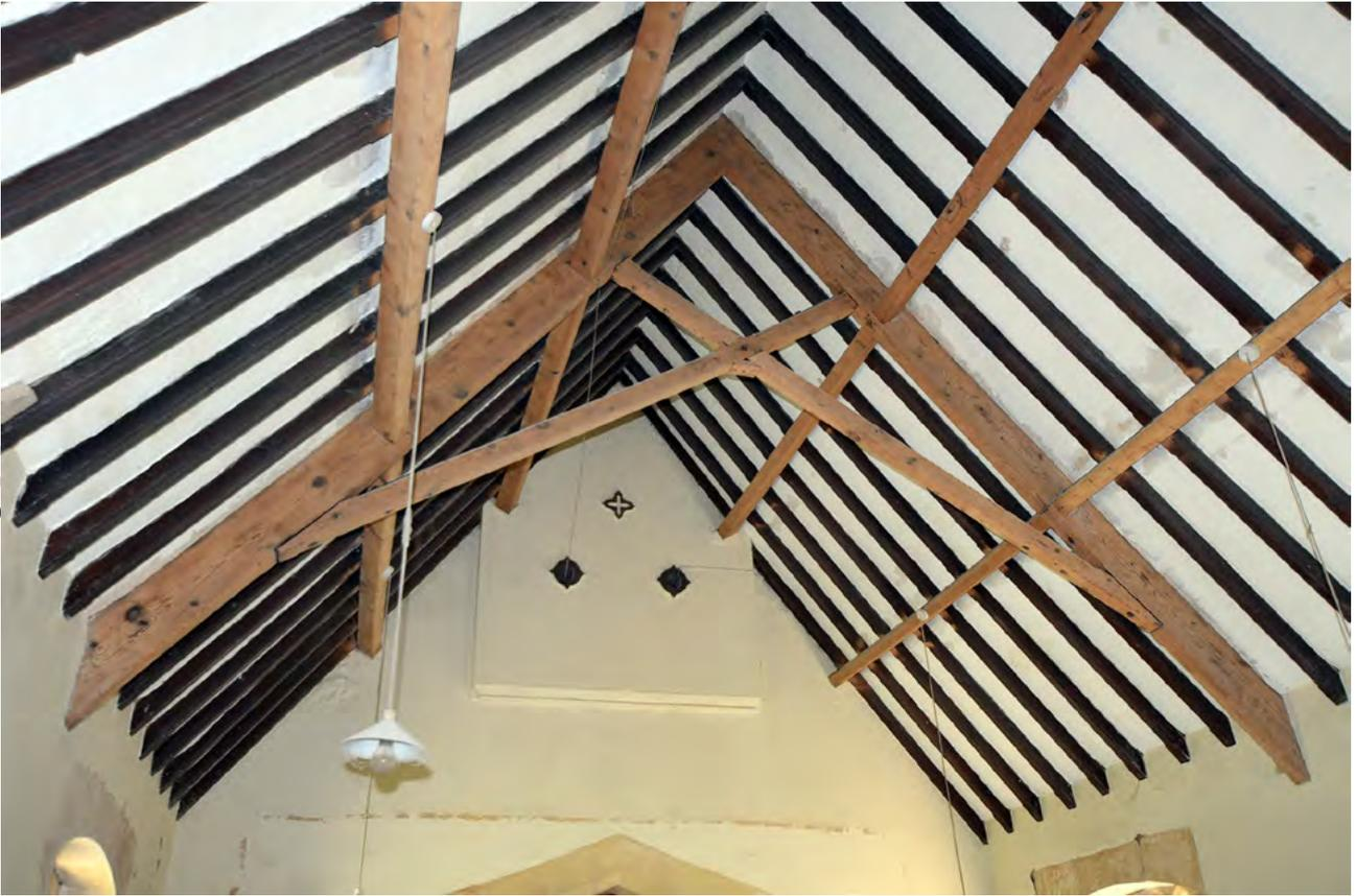
Plate 40: Scissor brace roof looking east
