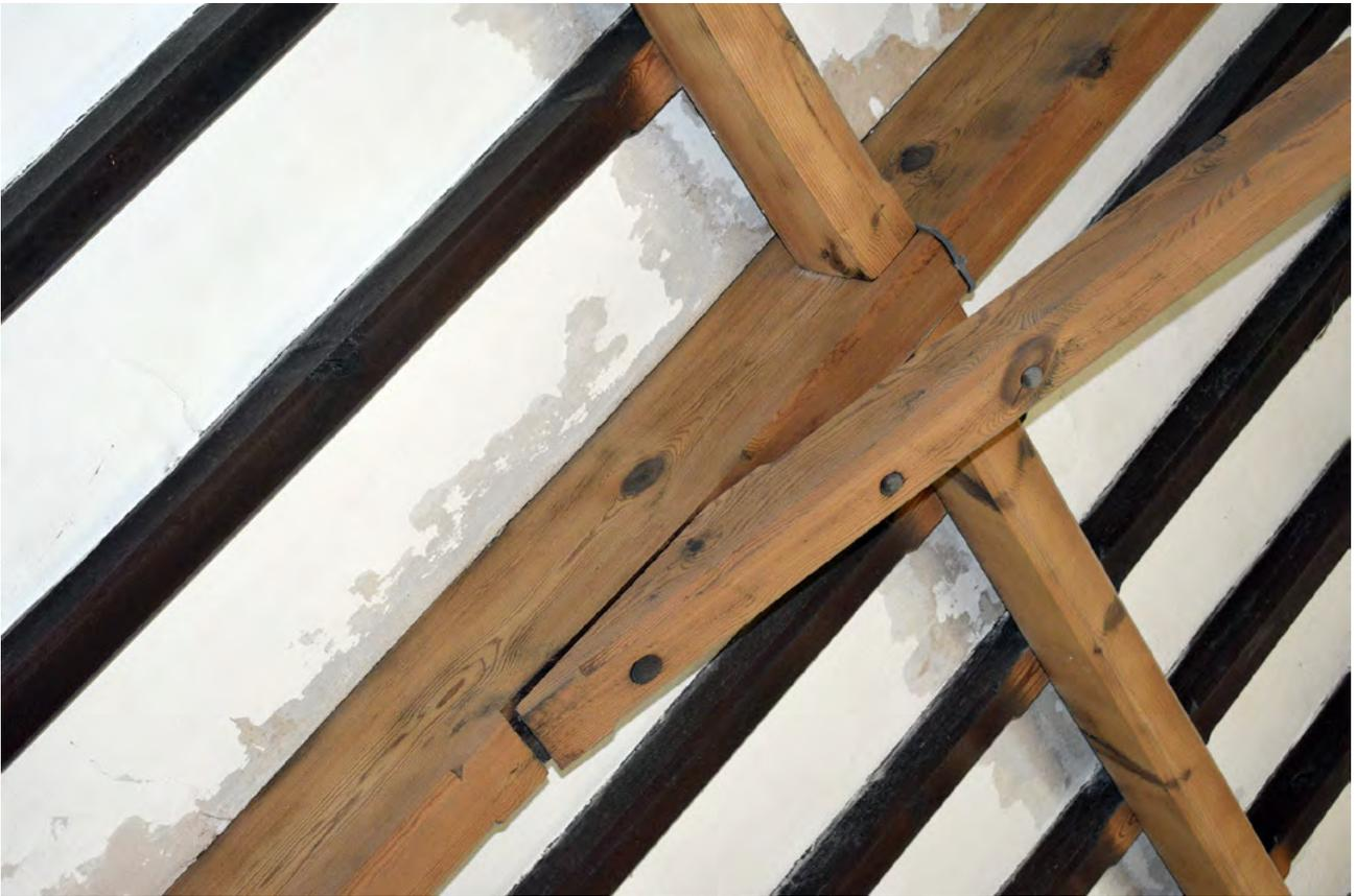
Plate 43: Detail of scissor brace roof
