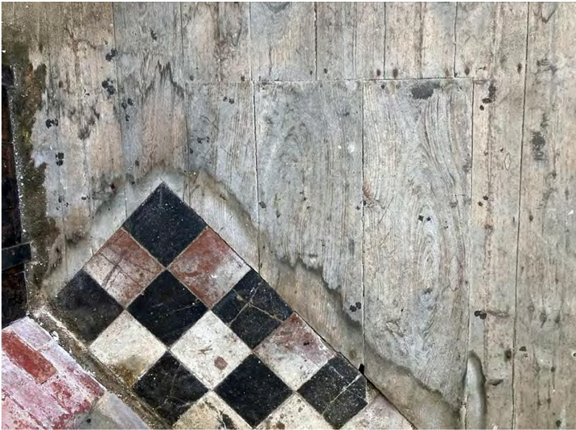
Plate 64: Small section of surviving primary floorboards by fireplace hearth (photo provided by Geoff Bolam)
