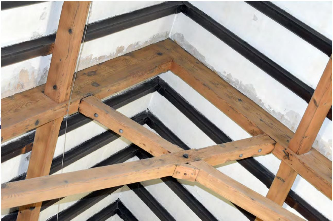
Plate 42: Detail of scissor brace roof
