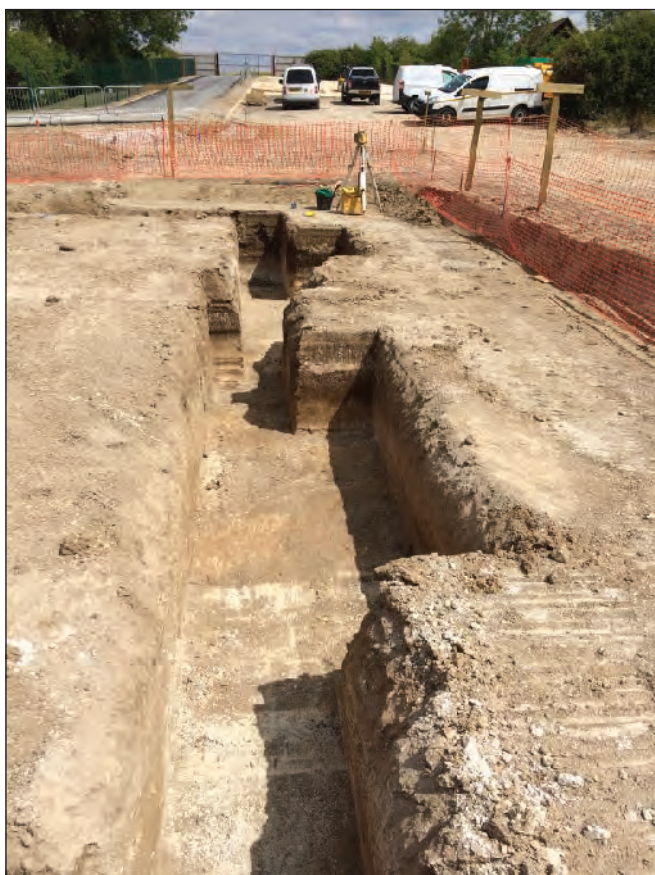
Plate 7: Strip foundations of house, clearly excavated below archaeological horizon into the natural geological chalk, looking east northeast
