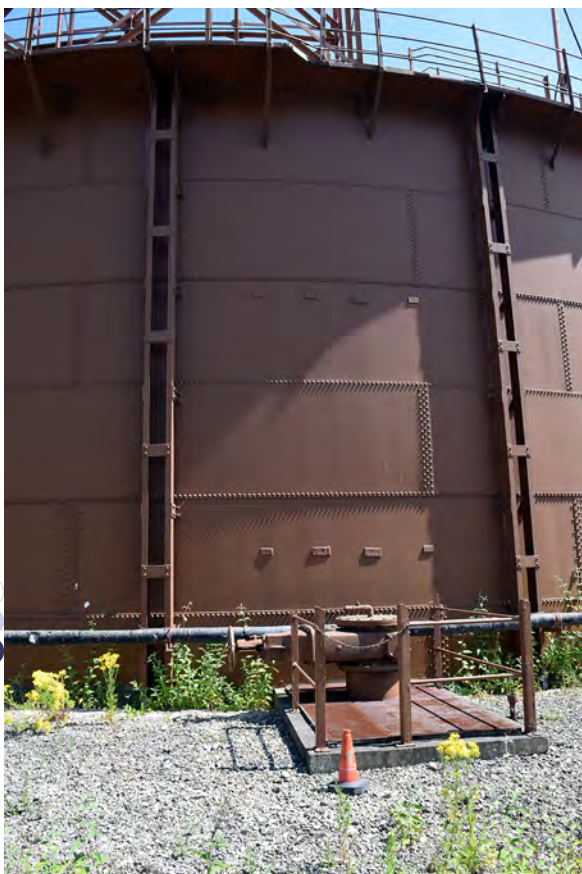
Plate 34: The disused dry well and remnants of removed brackets of Gasholder 2
