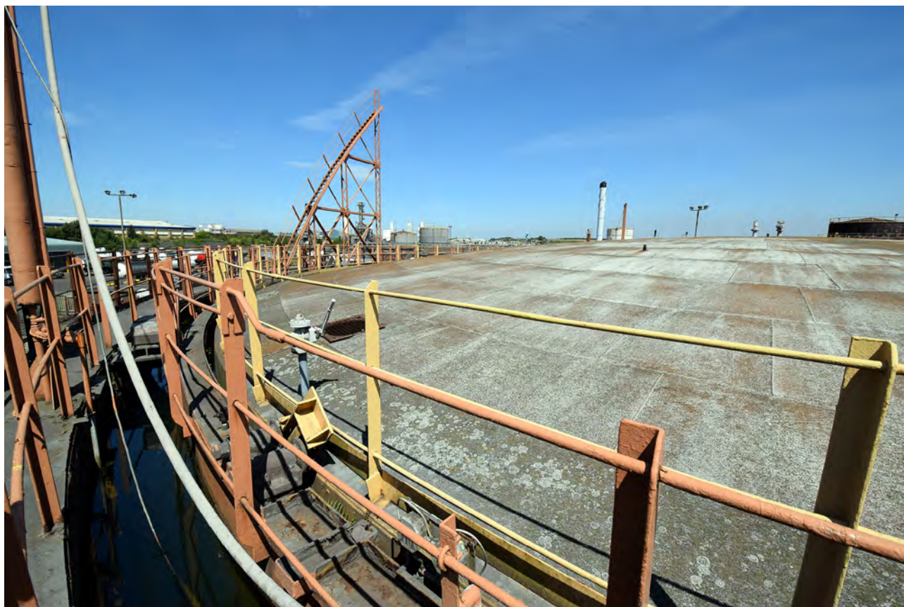
Plate 9: The crown of Gasholder 1
