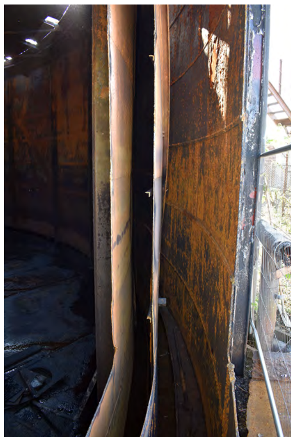
Plate 21: A section though the tank and lifts of Gasholder 1
