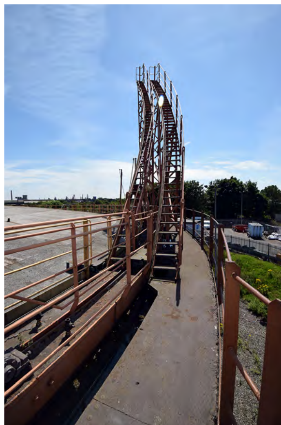
Plate 33: An example of the lift steps of Gasholder 2
