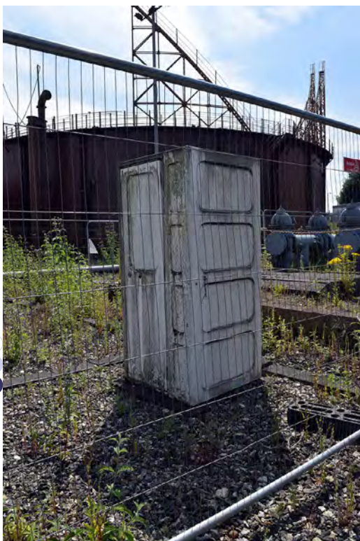
Plate 5: The telemetry kiosk within the distribution plant
