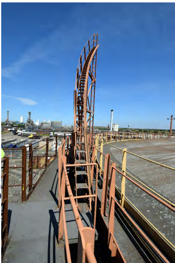
Plate 12: An example of the lift steps of Gasholder 1
