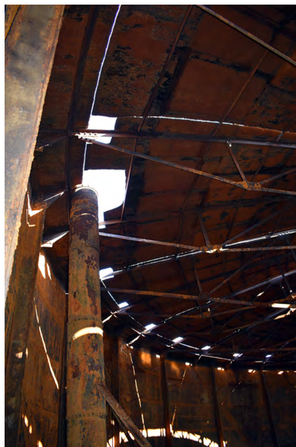
Plate 26: One of the inlet and outlet pipes in Gasholder 1
