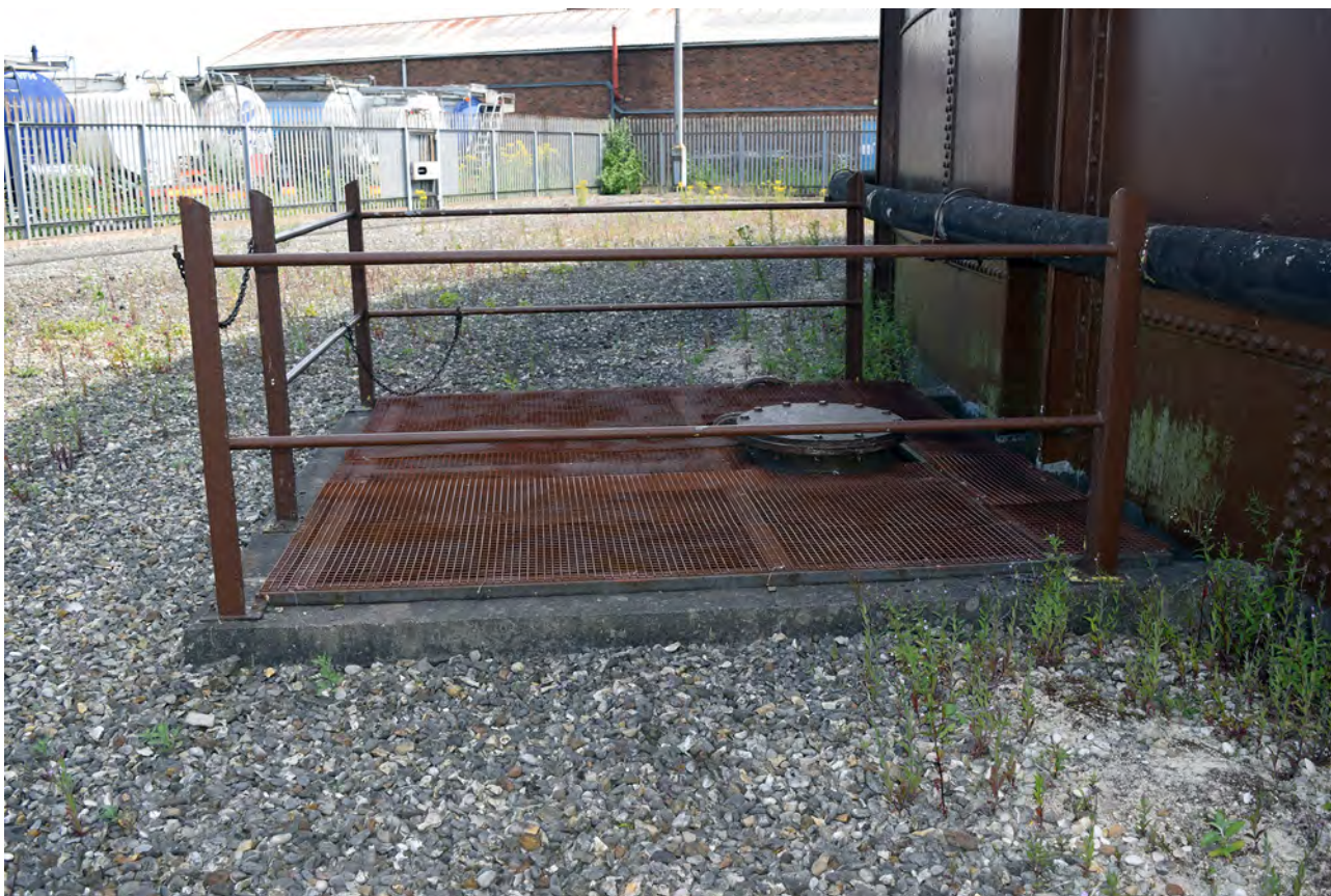
Plate 14: The covered disused dry well of Gasholder 1
