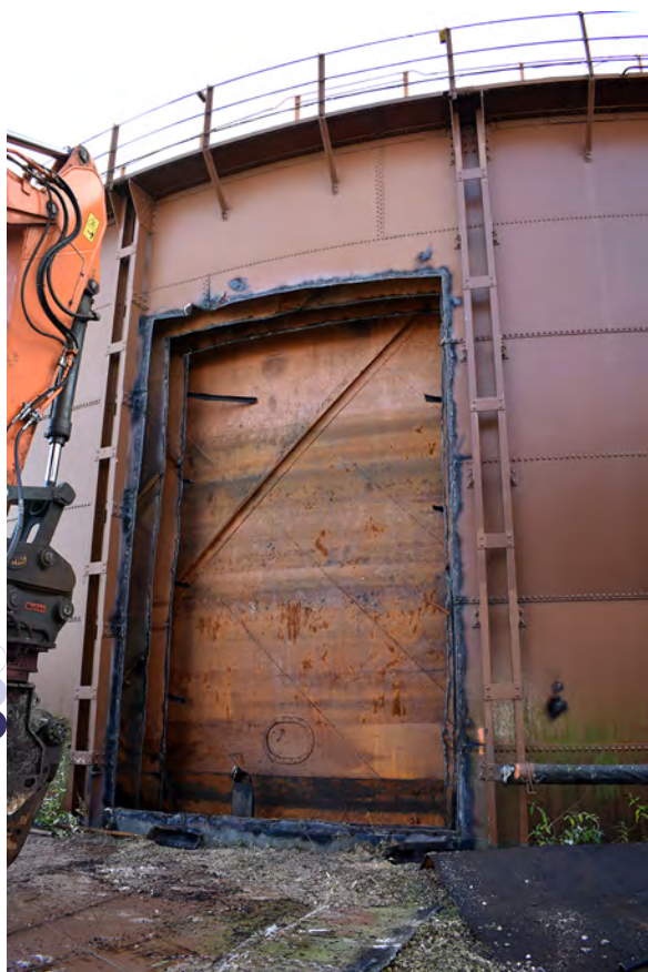
Plate 39: The opening being cut through Gasholder 2, looking south
