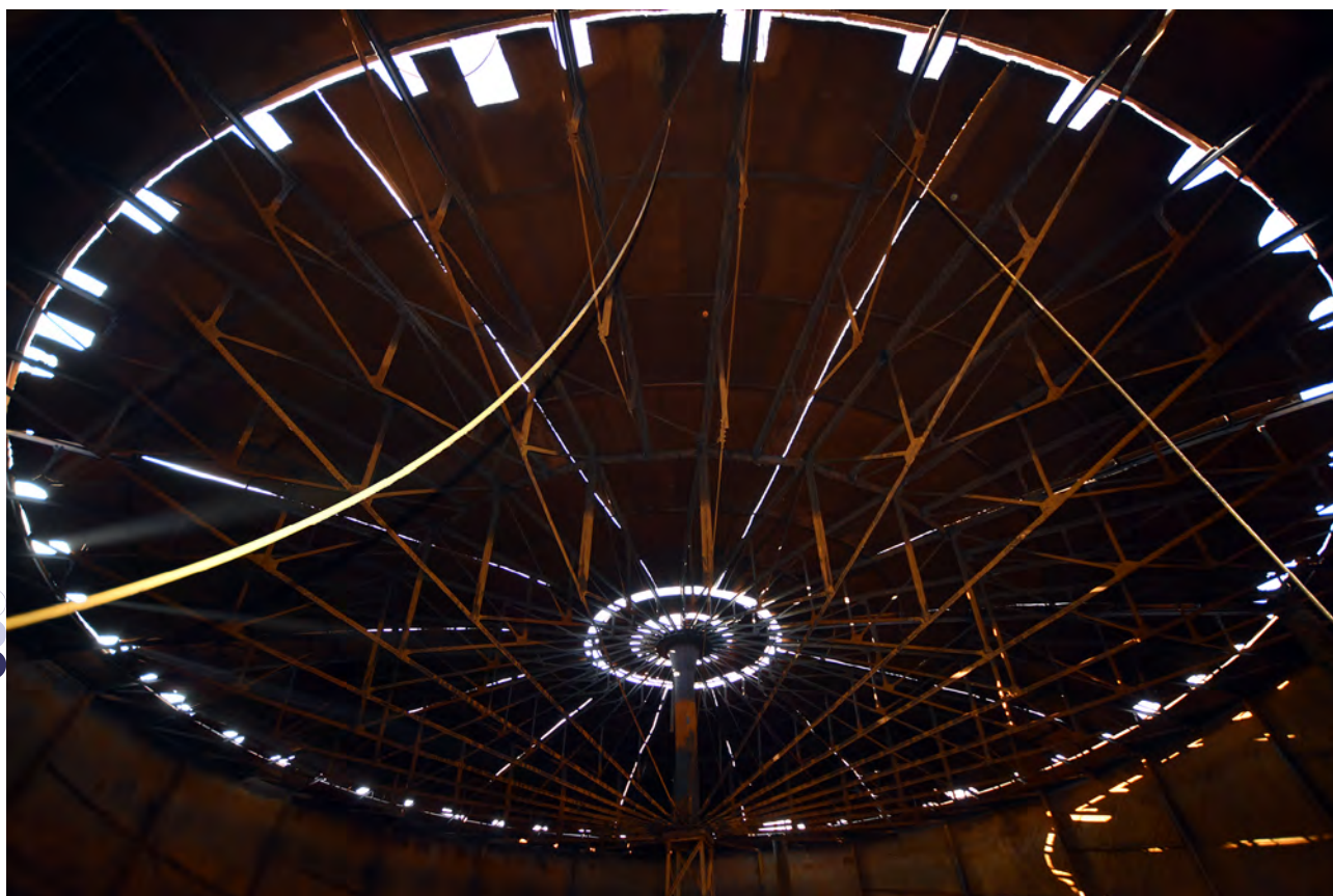
Plate 43: The crown structure of Gasholder 2
