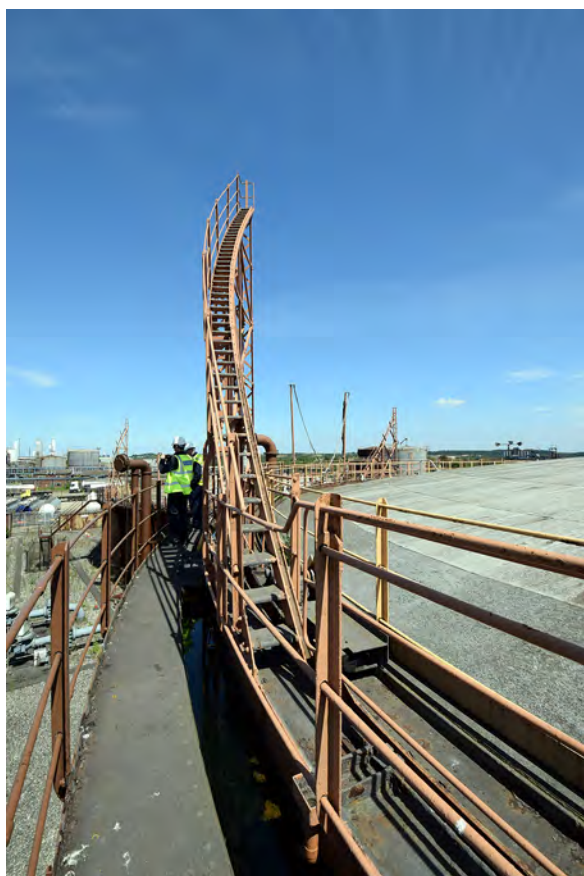
Plate 32: An example of the lift steps of Gasholder 2
