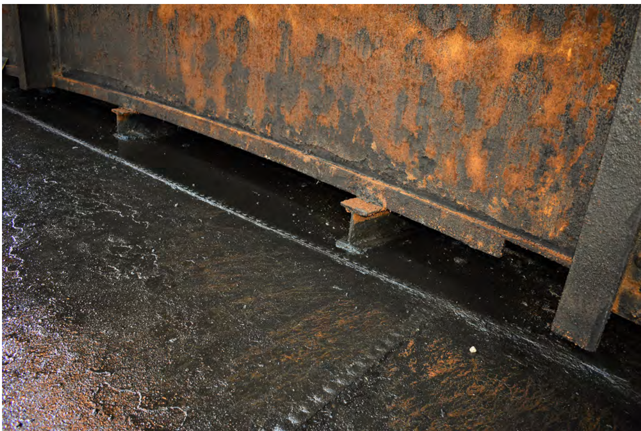
Plate 48: The supports at the base of the inner lift of Gasholder 2
