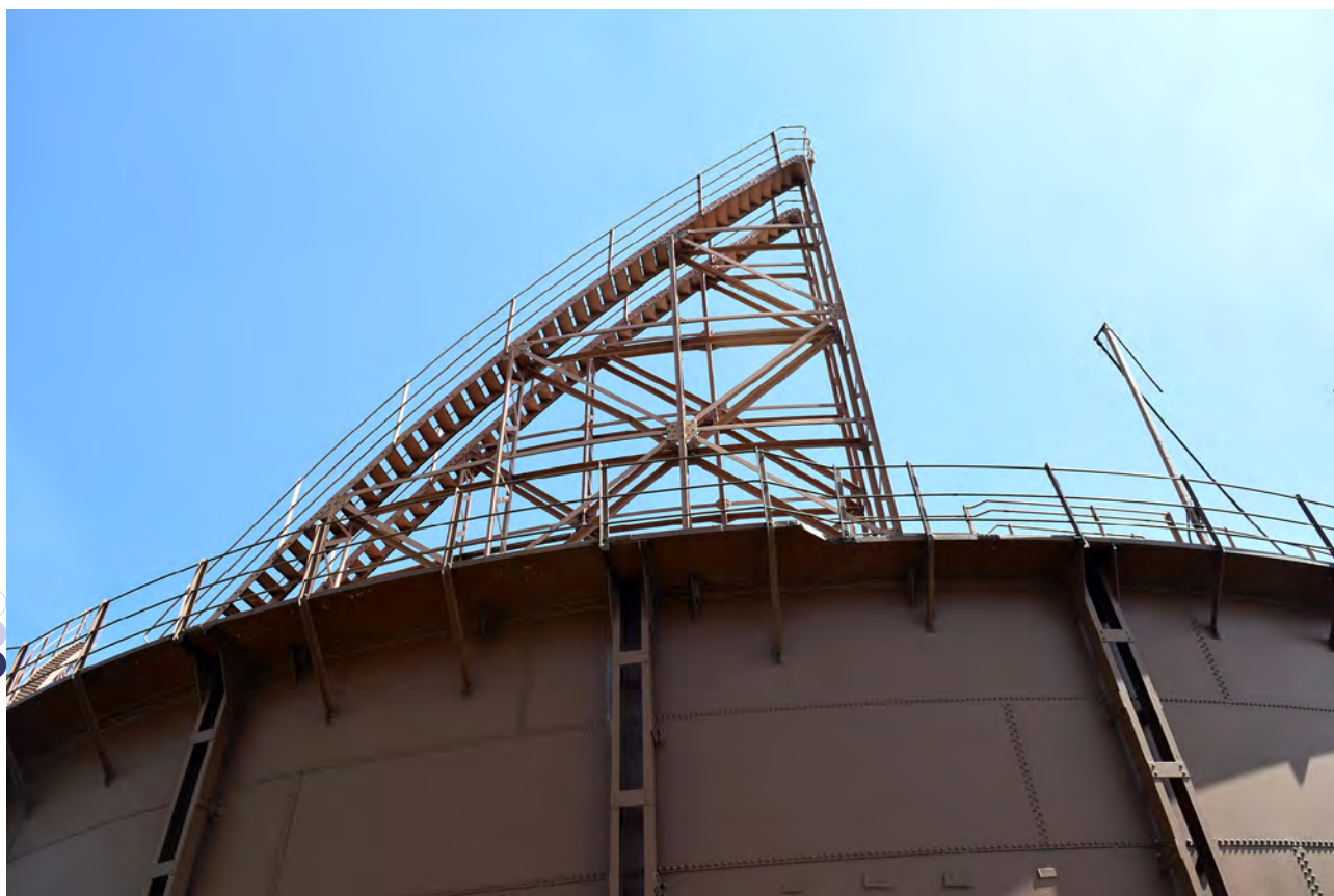
Plate 31: An example of the lift steps of Gasholder 2
