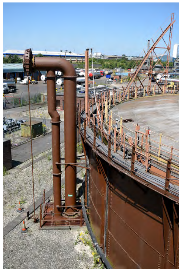
Plate 13: The inlet and outlet pipes and the anti-freeze system of Gasholder 1
