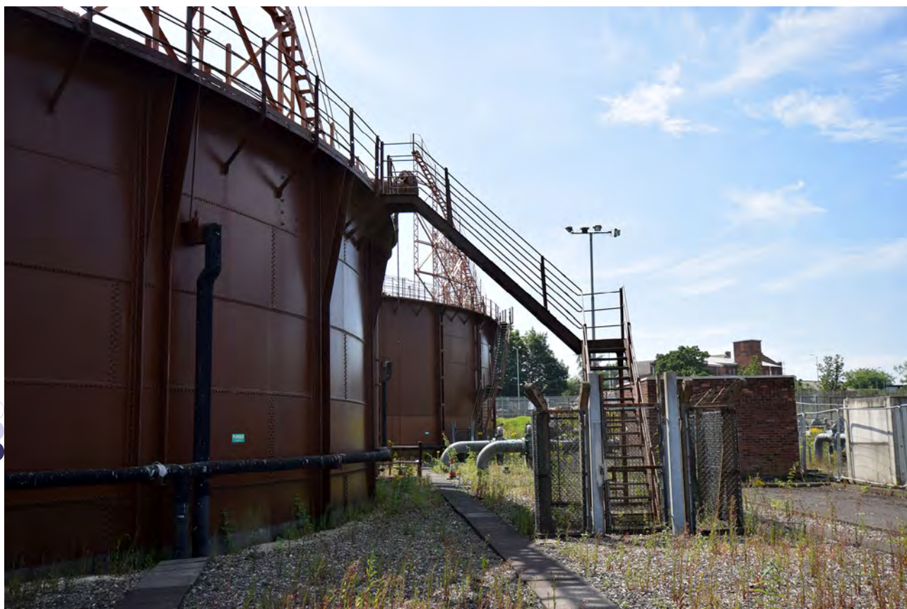
Plate 15: The off-set staircase of Gasholder 1
