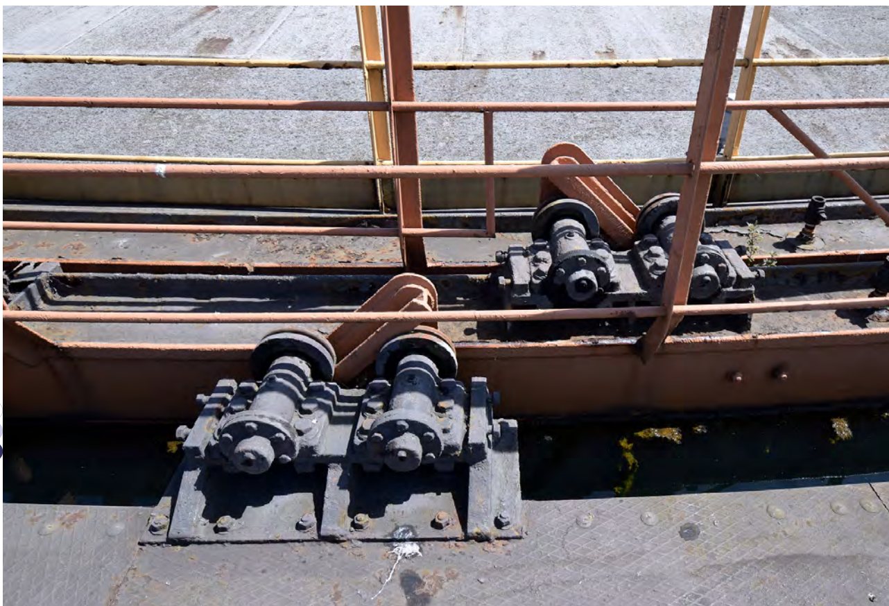
Plate 37: An example of the roller carriages of Gasholder 2
