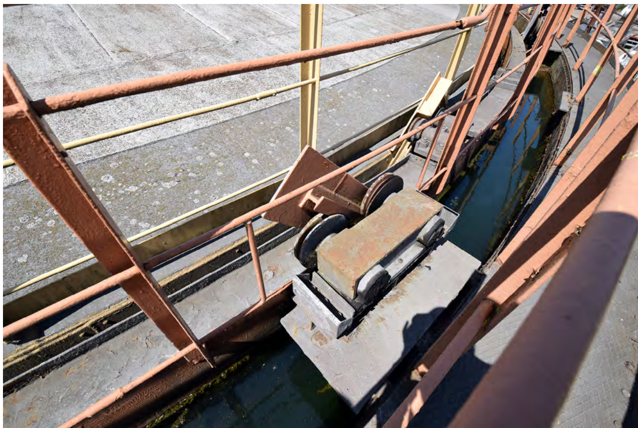
Plate 16: An example of the roller carriages of Gasholder 1
