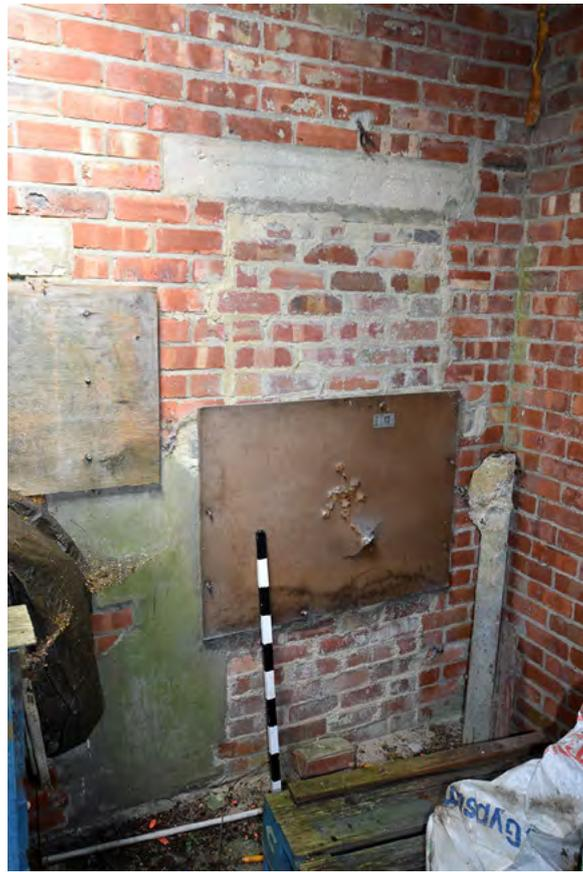
Plate 36: Blocked doorway at east end of north wall in Building 5
