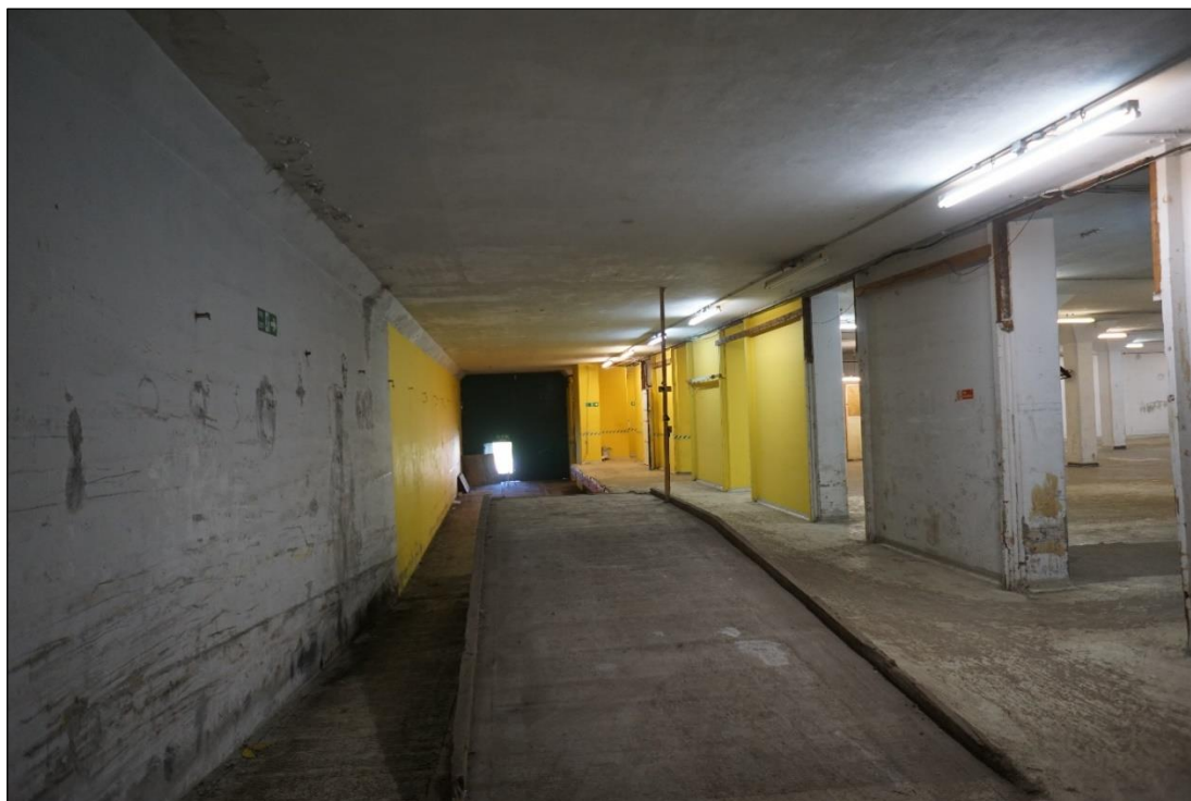
Plate 13: Loading bay facing north, with ramp to centre, full height openings to right of frame and truncated brackets on the opposing wall
