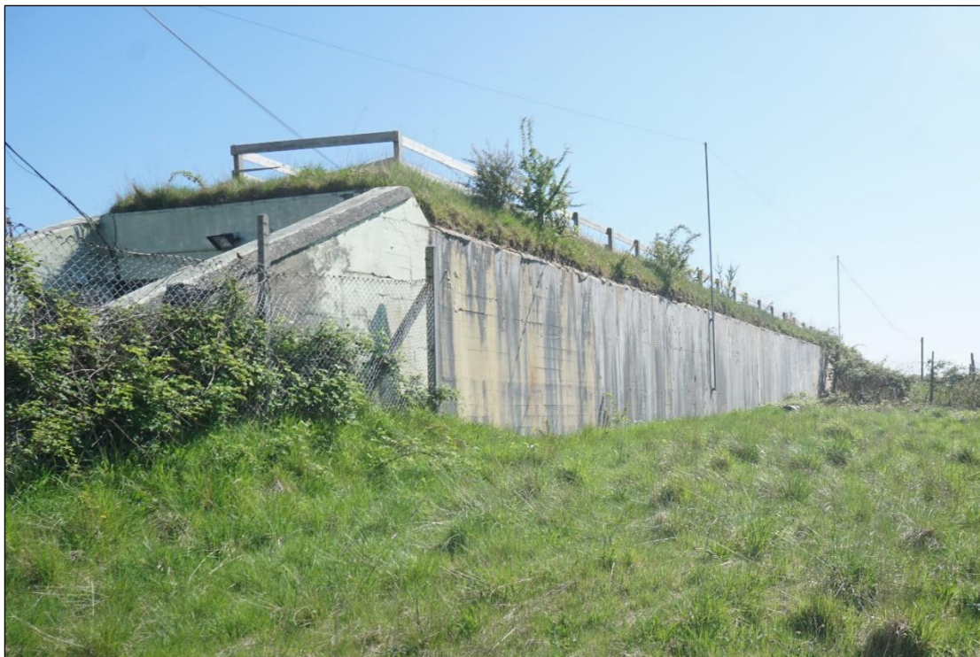
Plate 10: Western elevation, note the horizontal lines denoting the use of the cast in place technique
