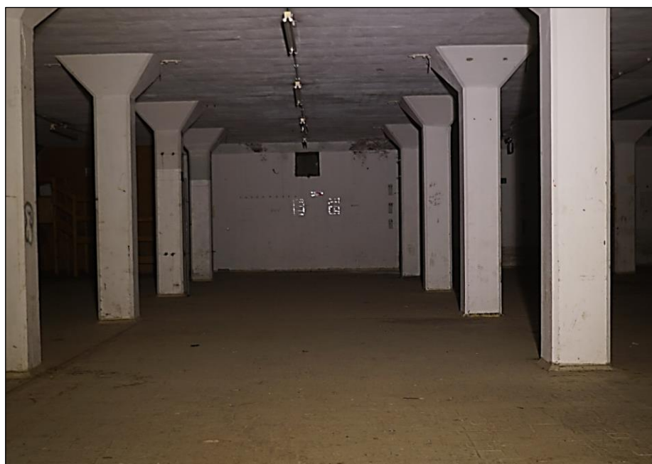
Plate 27: Penultimate northern bay, facing east. Note the square aperture in the eastern wall, one of two on this wall which coincides with the external ventilation towers
