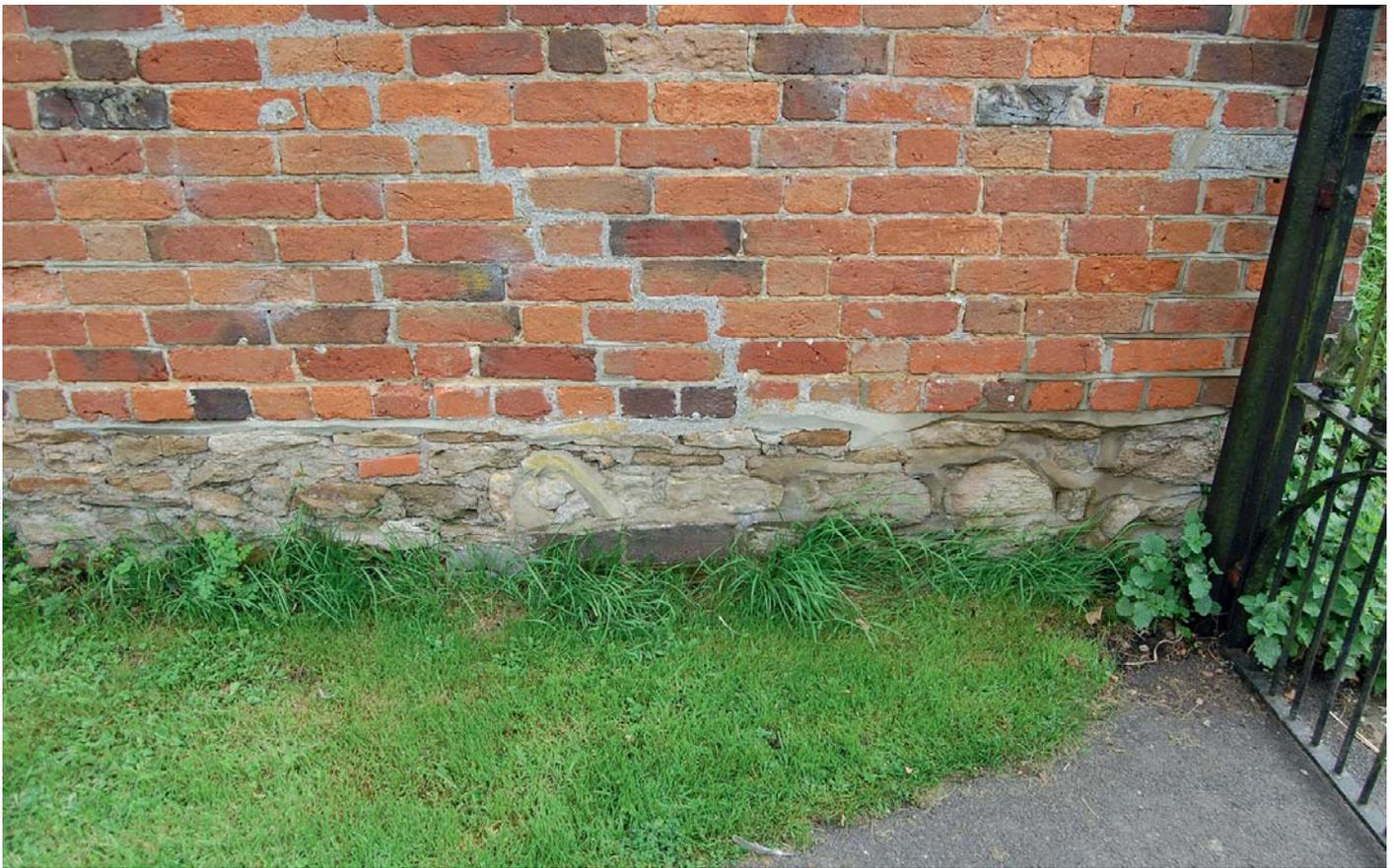
Plate 9 Repaired cracking in the west elevation
