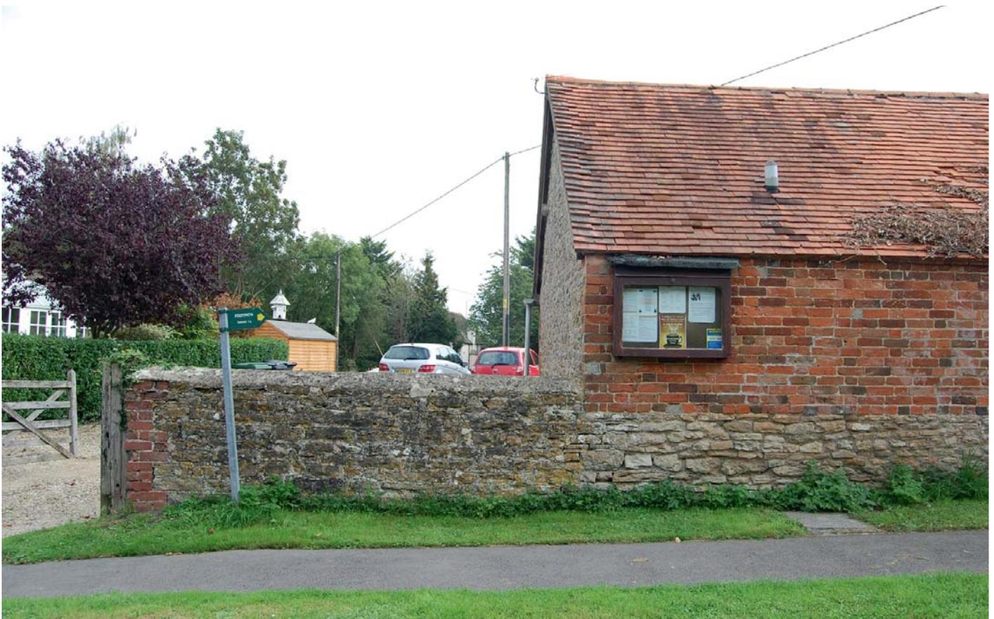
Plate 10 Limestone boundary wall abutting the barn
