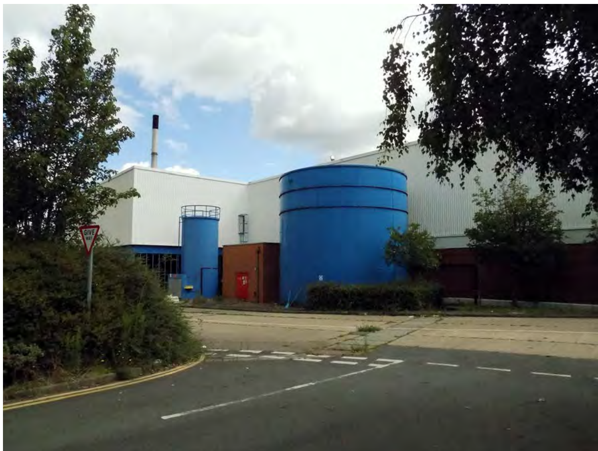
Plate 188: West side of new warehouse with pump room and water tank
