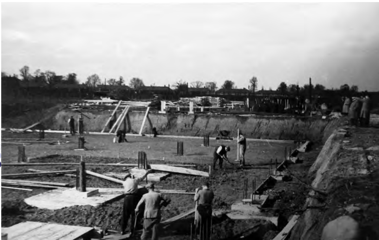
Appendix plate 3: View from the summer of 1936 showing the excavated basement for the new factory. Note column bases in the process of formation (from scrapbook of historic photographs found on site)
