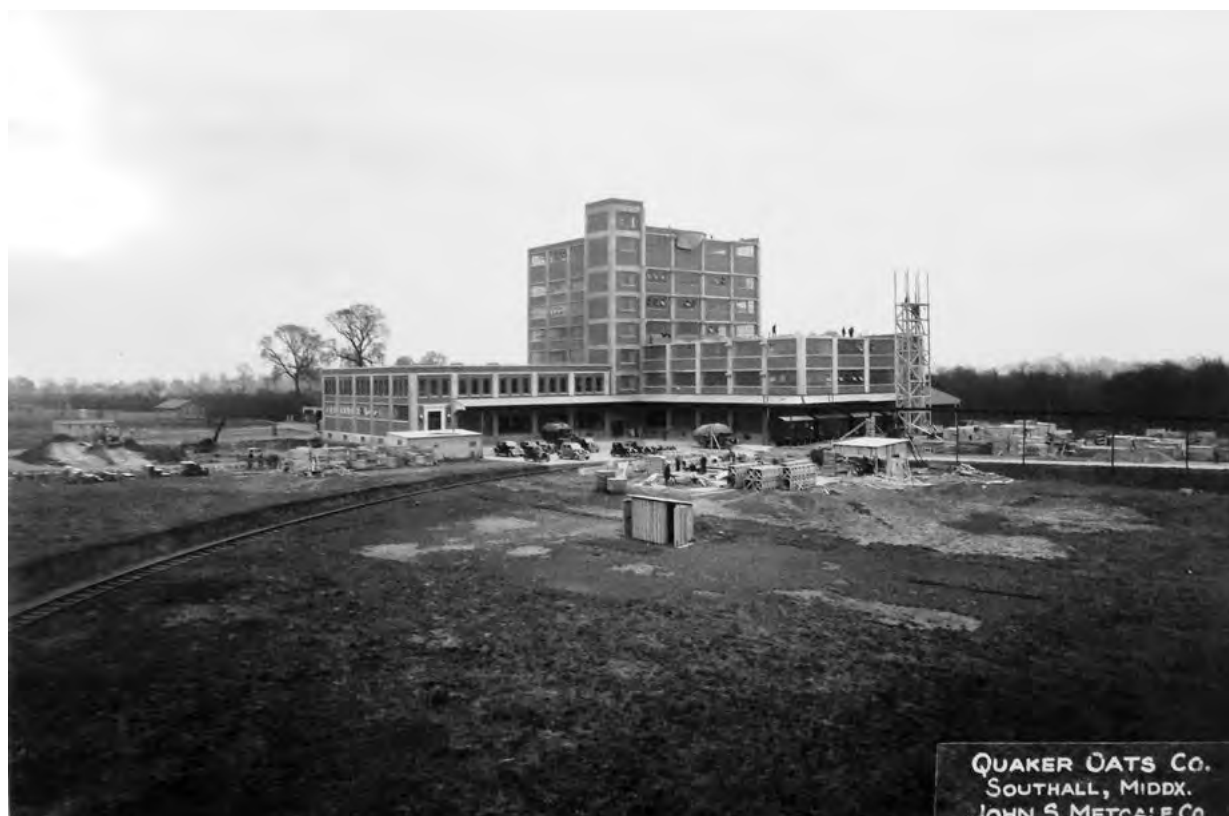
Appendix plate 5: View from north-west, dated 4 February 1938, showing the original form of Block A (centre and right) and Block B (left). The image also shows the start of works to raise Block A to seven storeys along its full length and to add a single storey extension to Block B (from scrapbook of historic photographs found on site)
