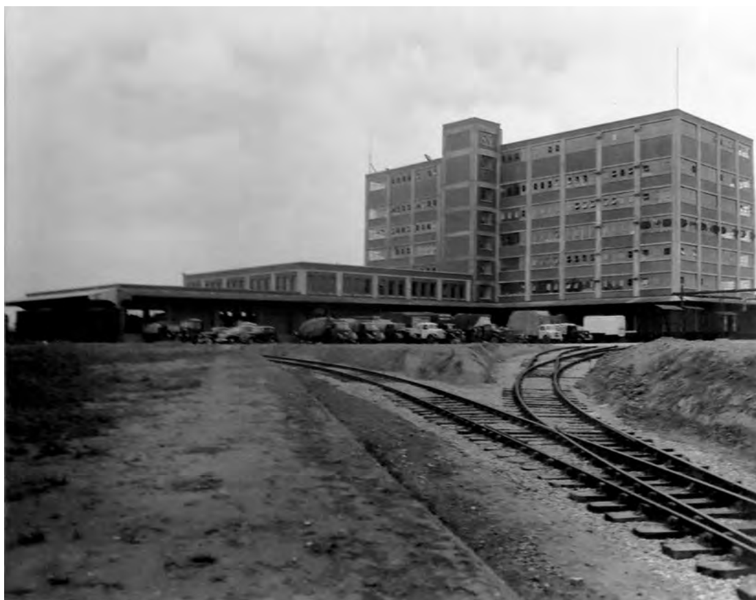
Appendix plate 8: View from south-east showing the additional rail sidings added in 1948 on the west side of Building A and the spur line to the north side of Building B (from scrapbook of historic photographs found on site)
