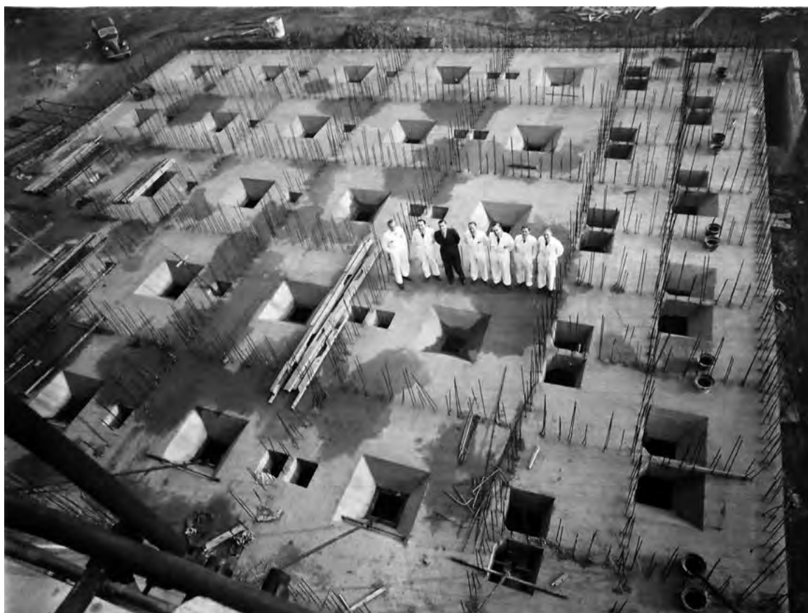
Appendix plate 13: View from May 1953 showing the base of the new silos range during its construction (from scrapbook of historic photographs found on site)
