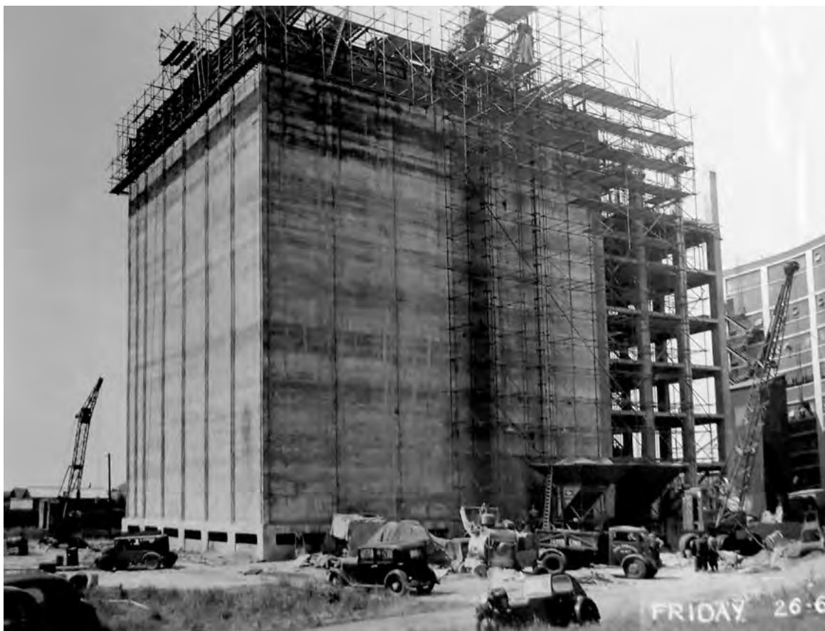
Appendix plate 16: Two images from June 1953 showing the continuous pouring process of constructing the silos (from scrapbook of historic photographs found on site)
