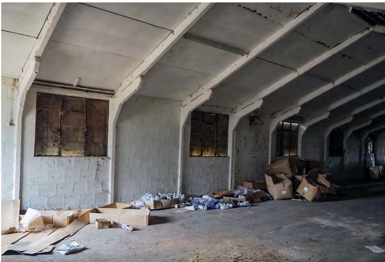
Plate 29: Building 10, internal view of portal frames and critted windows
