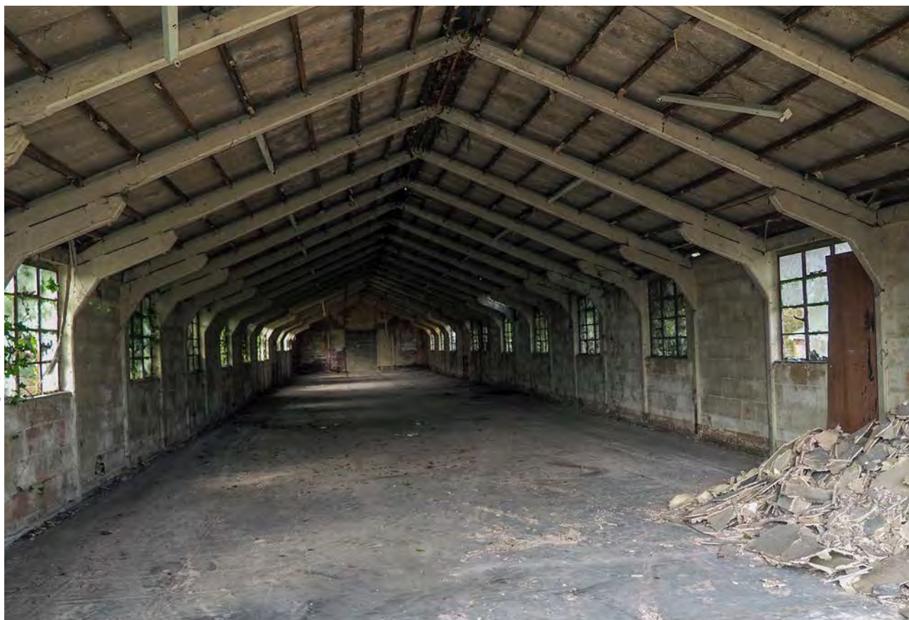
Plate 5: Building 24, internal view of portal frames
