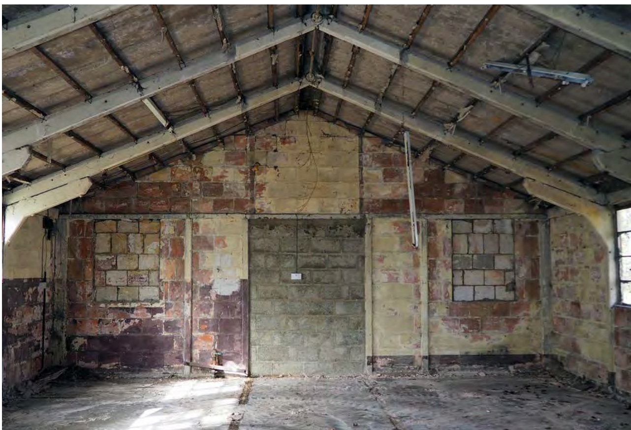
Plate 14: Building 24, internal view showing evidence of former room partitions
