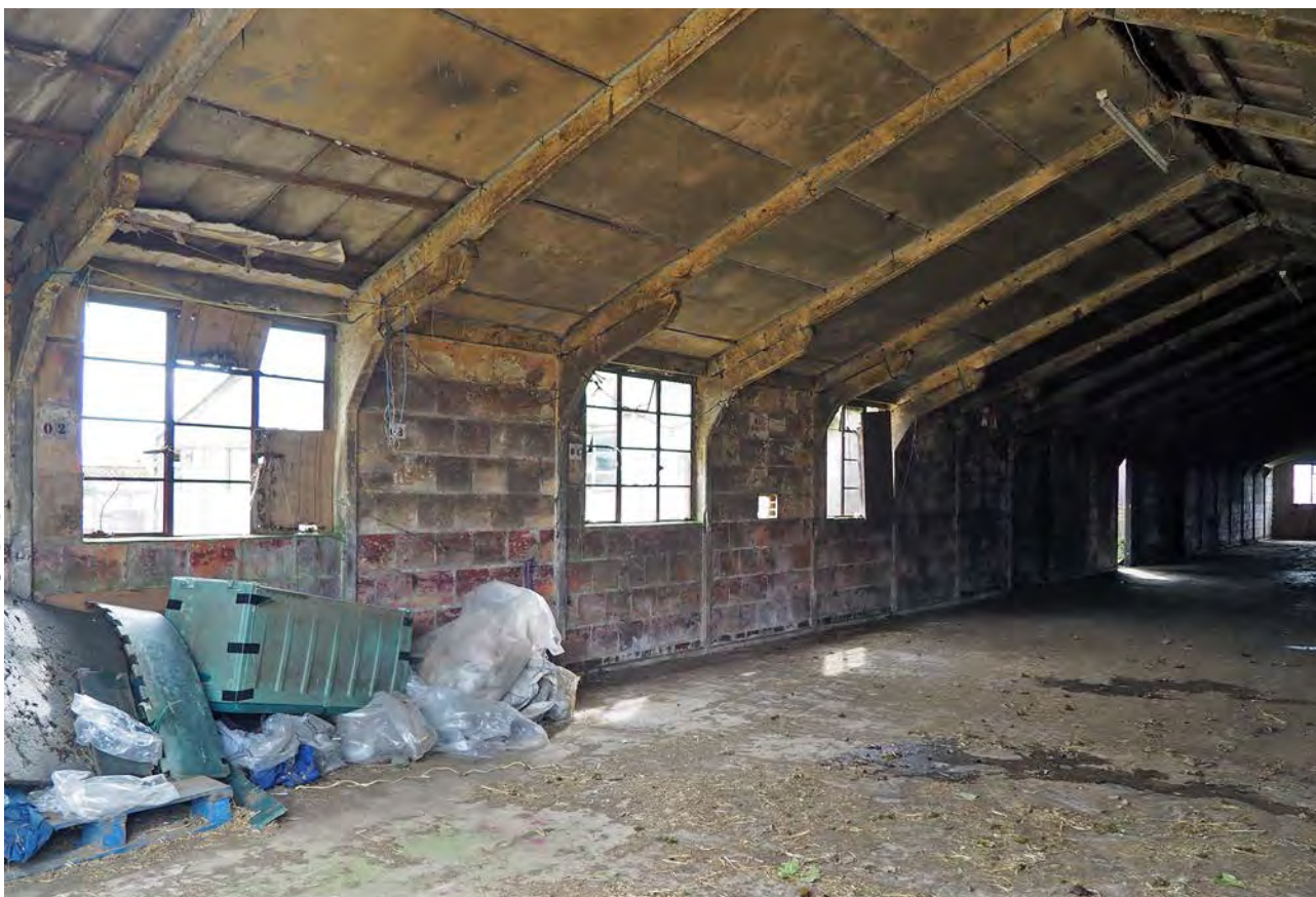
Plate 7: Building 17, hard board ceiling
