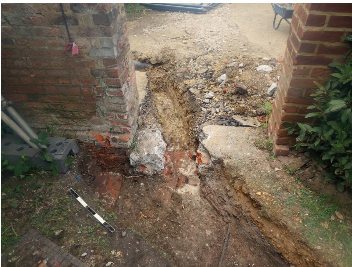
Plate 43: Entrance through garden wall 615 showing rebuilt ends supported by concrete threshold over brick foundation 599, with brick wall 600 at right angles, looking north-west
