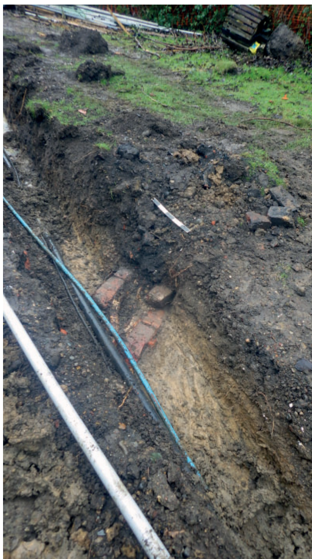
Plate 3: Brick conduit 458 section 69, looking south-west
