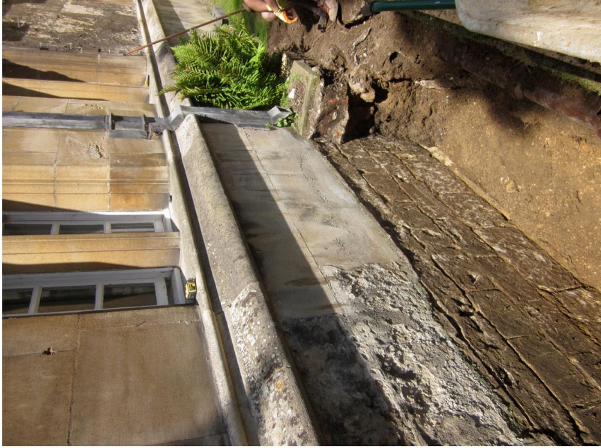
Plate 1: 1675-6 footing showing possible offset in base of trench
