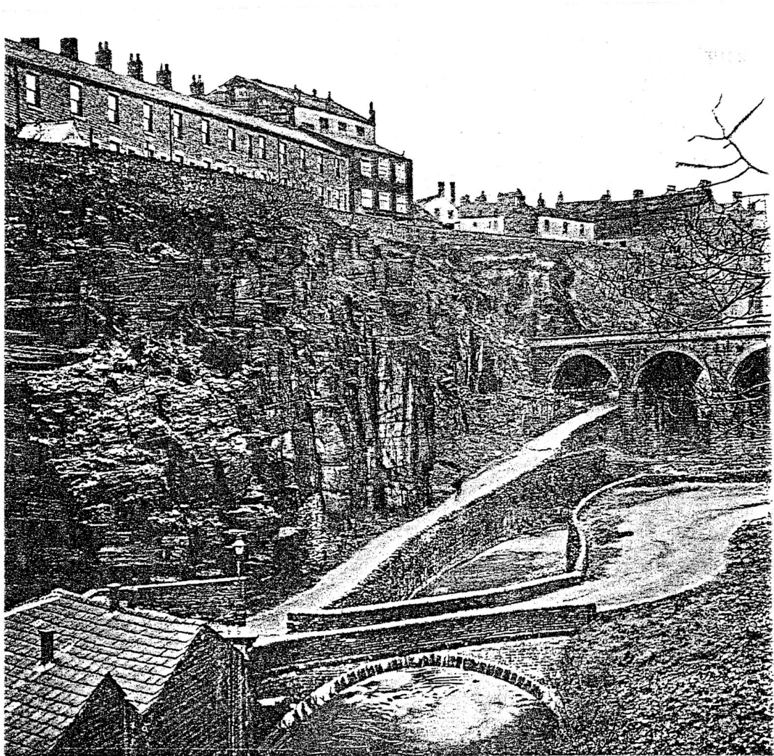
Plate 4: Railway viaduct (Site 12) and Torr Mill in the foreground
