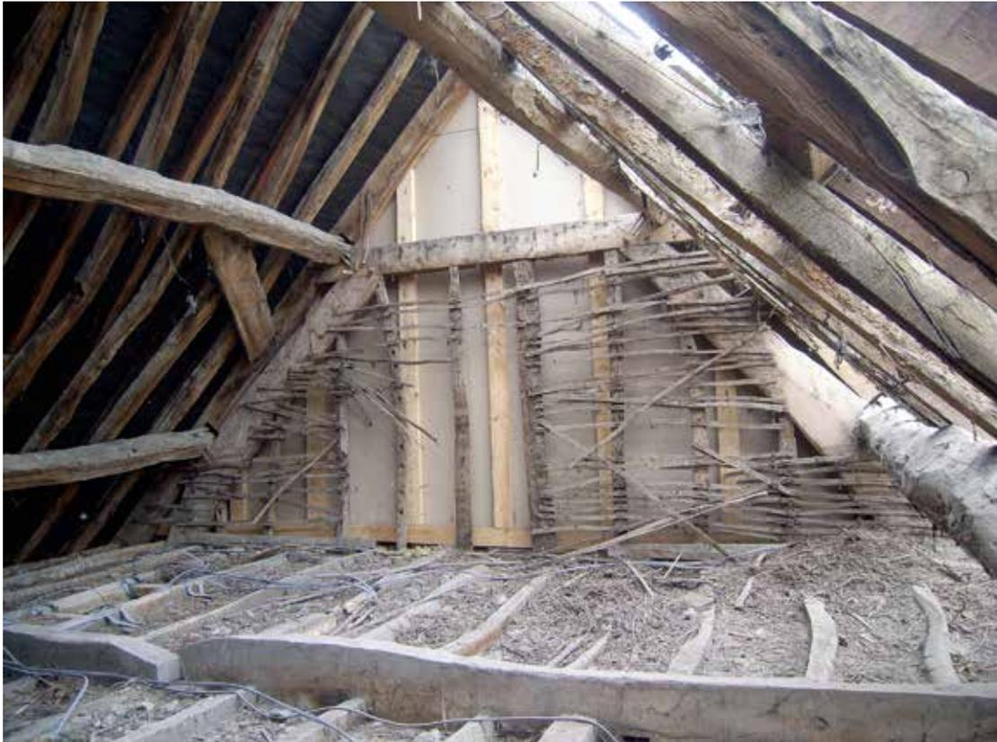
Plate 22 *Truss with clasped inner principals (No. 32–33)*
