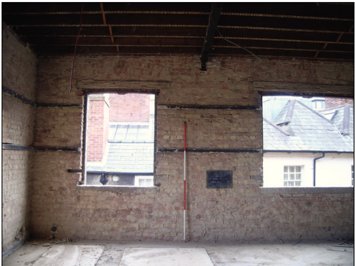
Plate 12: Interior showing lintels and relieving arches over windows and fixing timbers.
