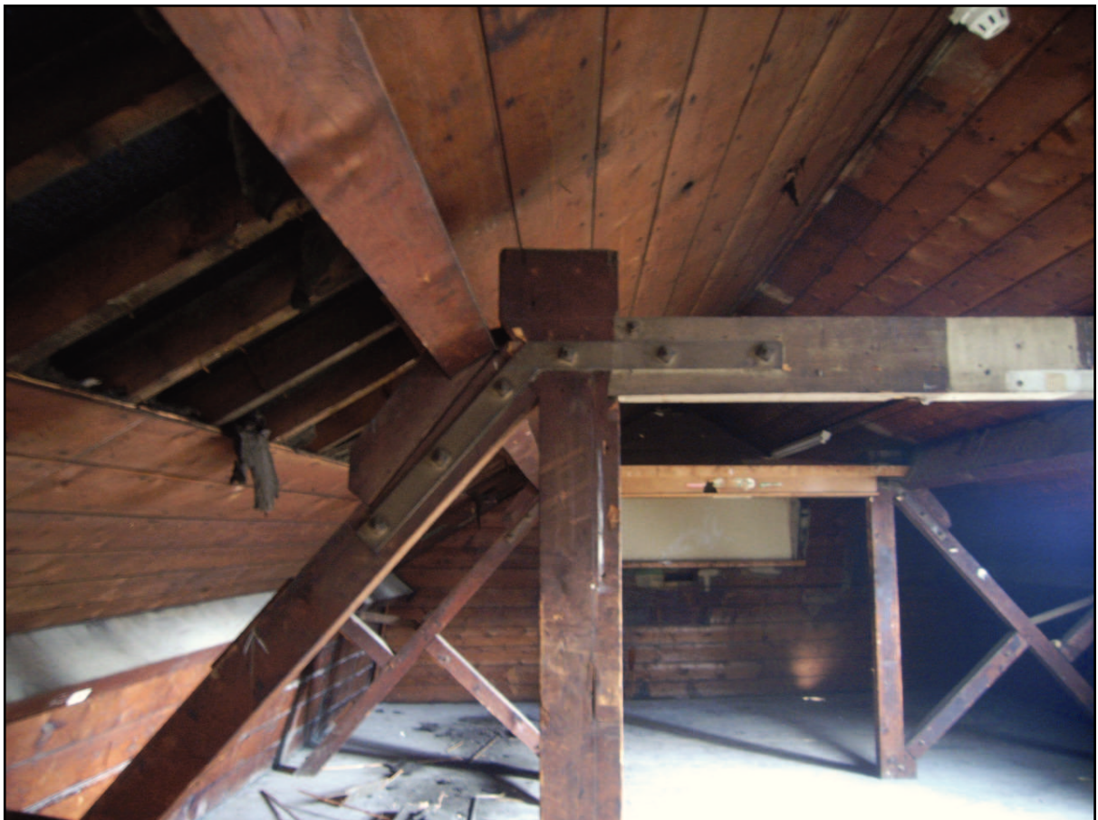
Plate 16: Detail of truss joint between principal rafter, strainer and queen post.
