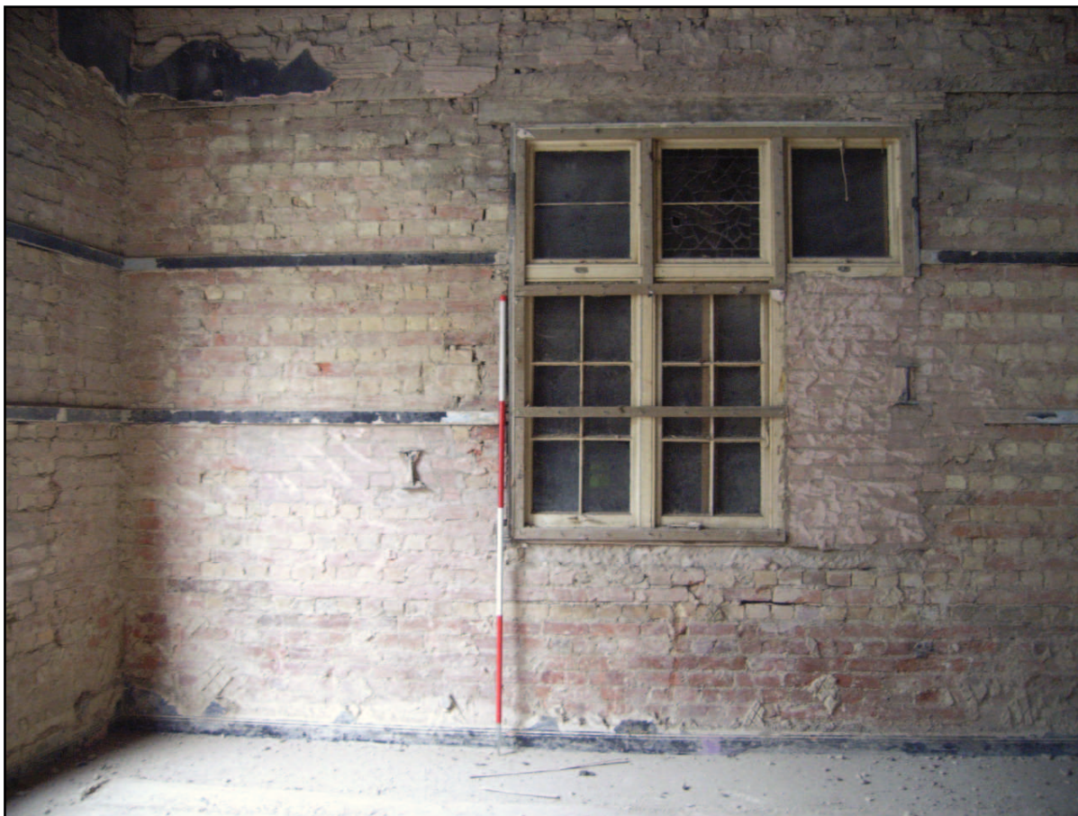
Plate 13: Surviving primary window at west end of first floor.
