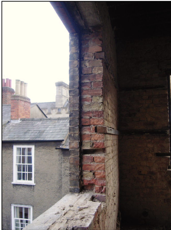
Plate 11: Jamb of window opening showing detail of wall construction.
