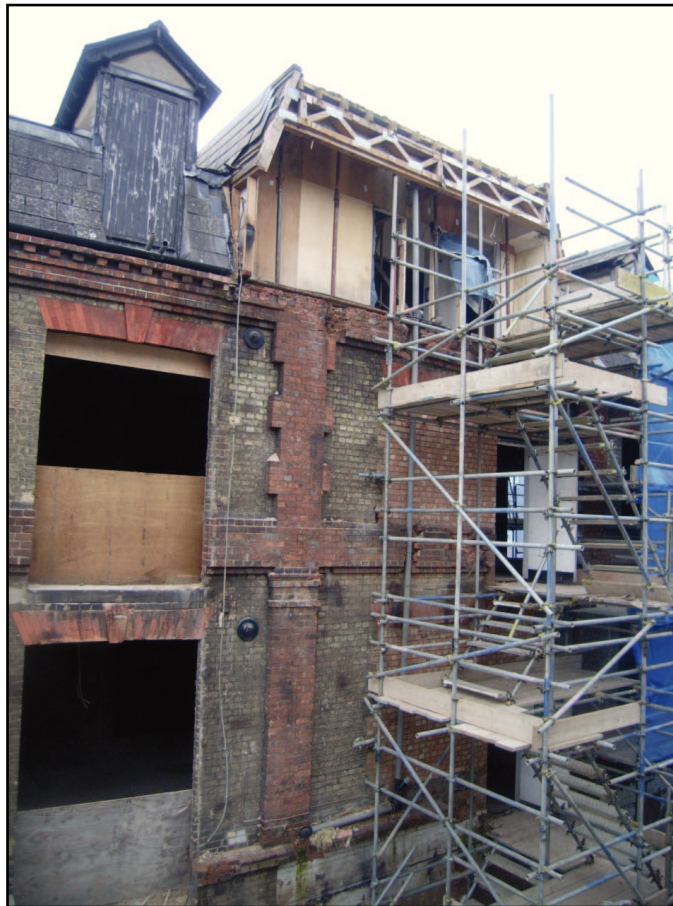
Plate 7: Third and fourth bays from west on south side showing door in dormer and door openings below, blocked former windows and remnant of extension roof.
