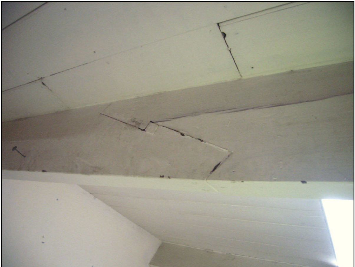
Plate 18: Splayed, tabled, keyed and under-squinted scarf joint in purlin
