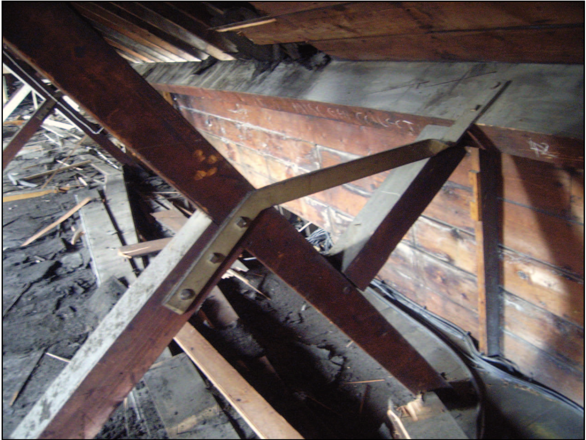
Plate 17: Detail of truss construction showing brace and strap supporting lower purlin.
