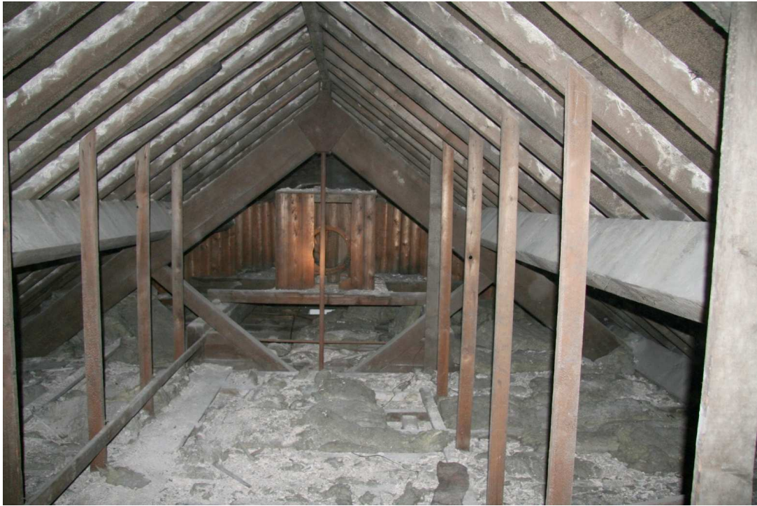
Plate 23: The roof structure above the main school building showing a truss and the box of the clock mechanism beyond
