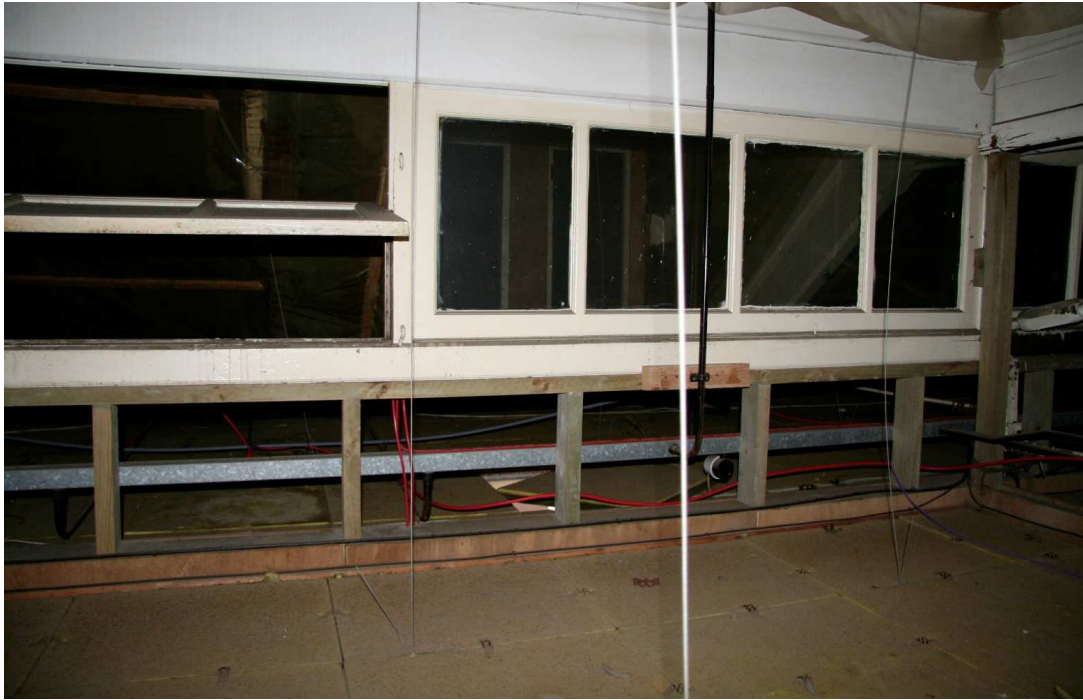
Plate 21: The line of original partitions preserved above suspended ceilings between the upper five class rooms and corridor Room 28
