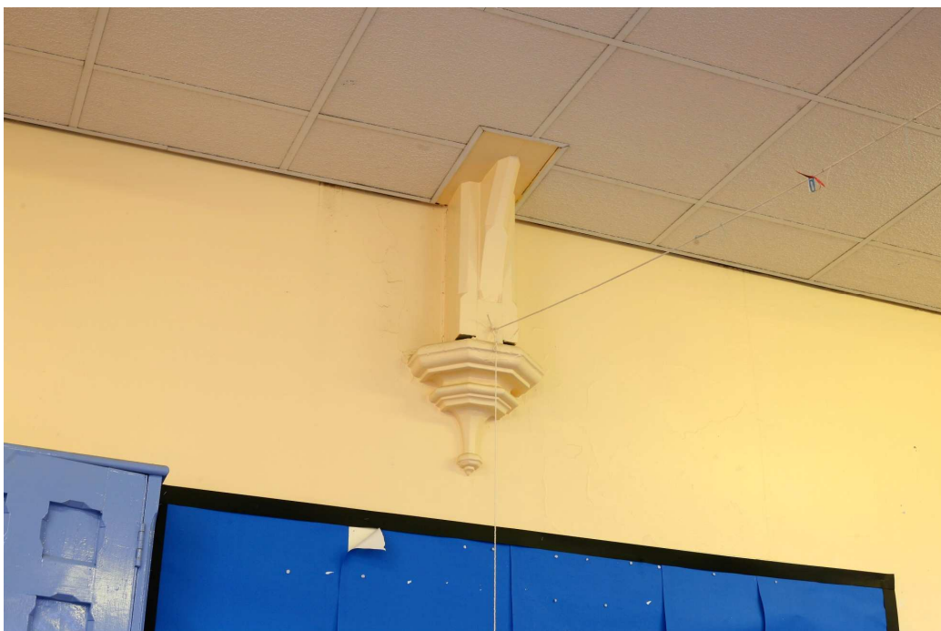
Plate 16: The wall plate and braces of a hammerbeam truss in Room 1
