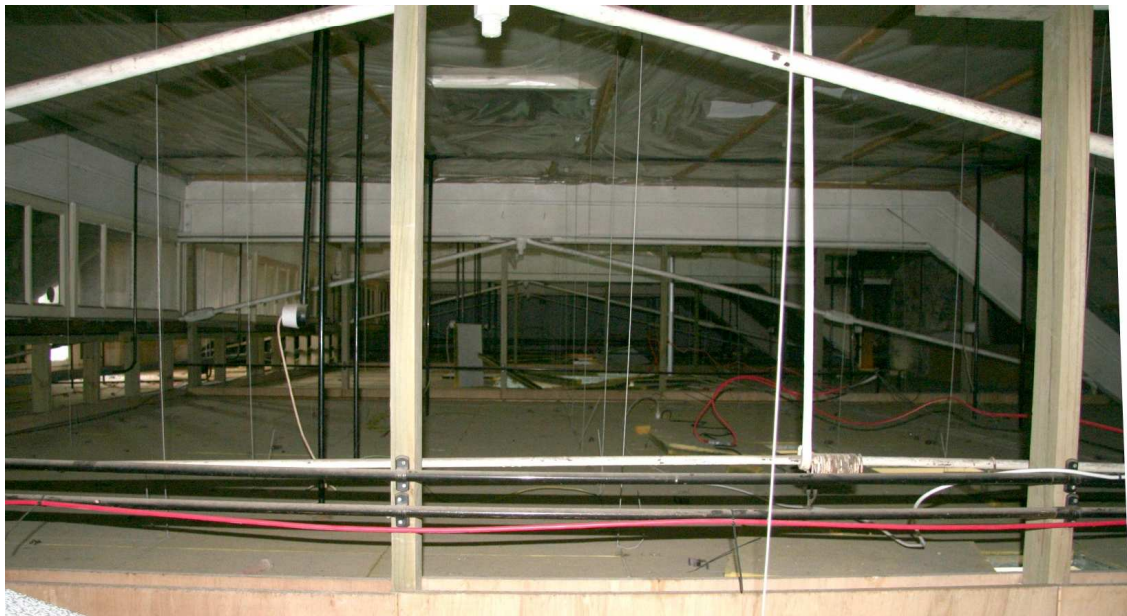
Plate 22: The lower part of a main school building truss preserved above a suspended ceiling, showing tie rods supporting the principal rafters
