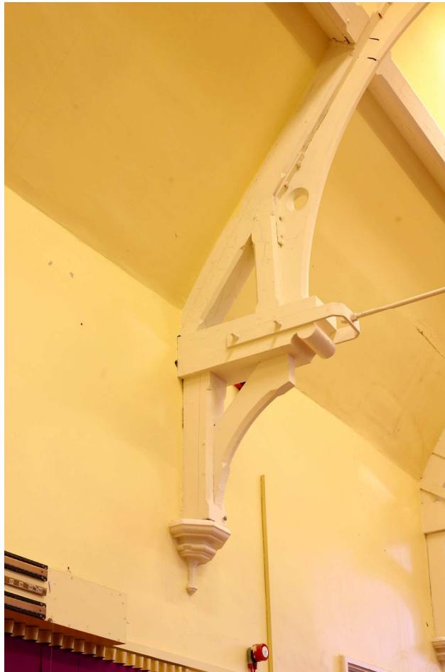
Plate 15: The wall plates and braces of the hammerbeam truss in Room 4
