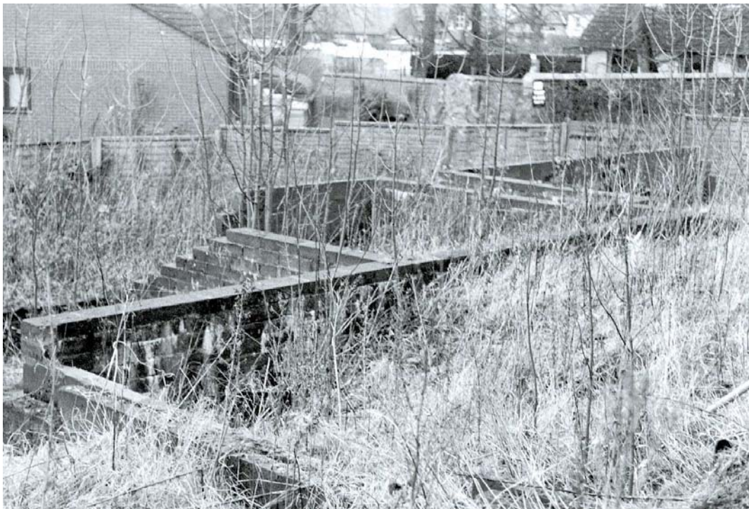
Plate 2: Site 27, in the north-eastern part of the site, looking north
