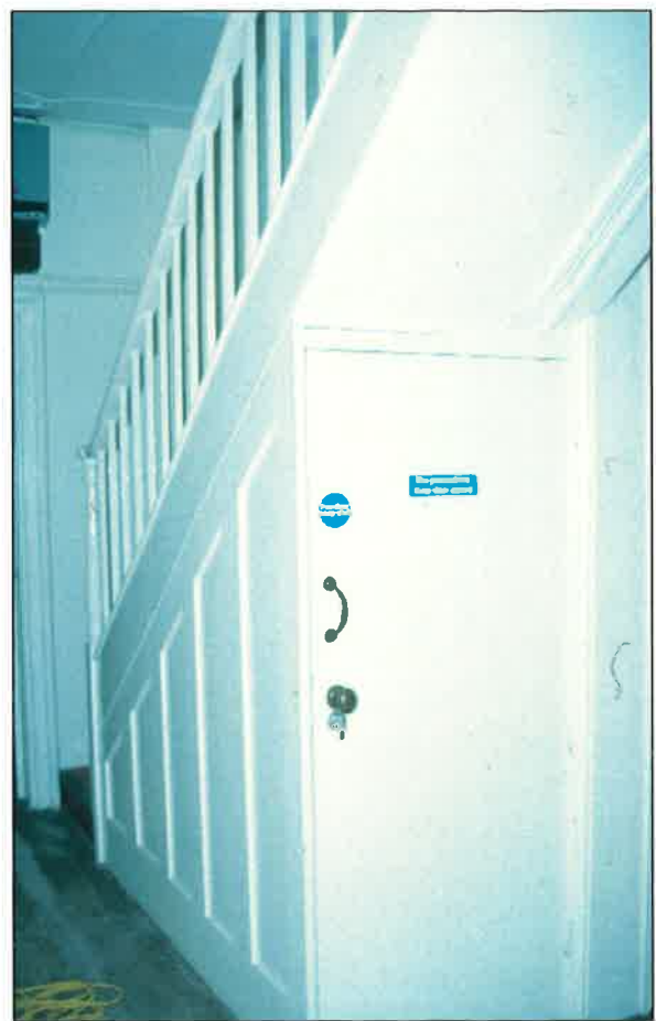
Plate 8: Staircase, ground floor
