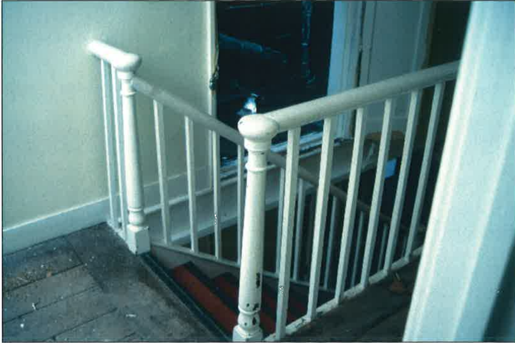
Plate 12: Staircase, second floor
