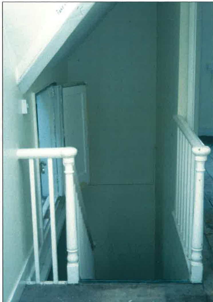
Plate 13: Staircase, second floor
