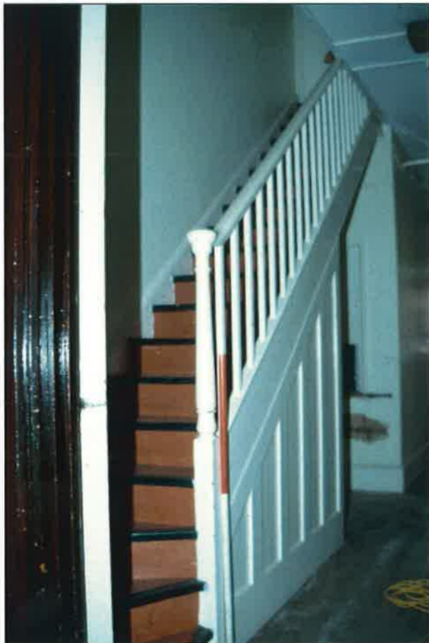
Plate 7: Staircase, ground floor
