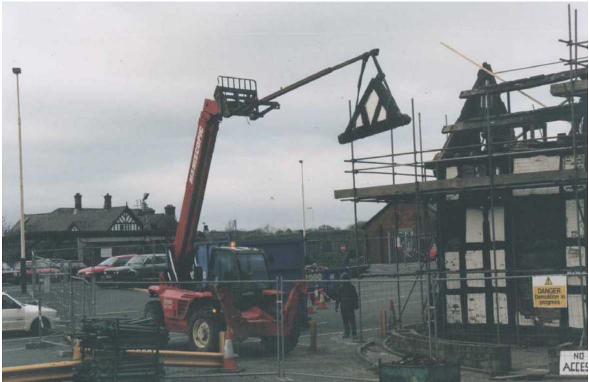
Fig 32: The dismantling of the West Wing timber frame
