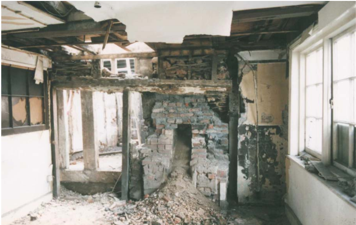
Fig 28 East External wall of the West Wing showing the Inglenook
