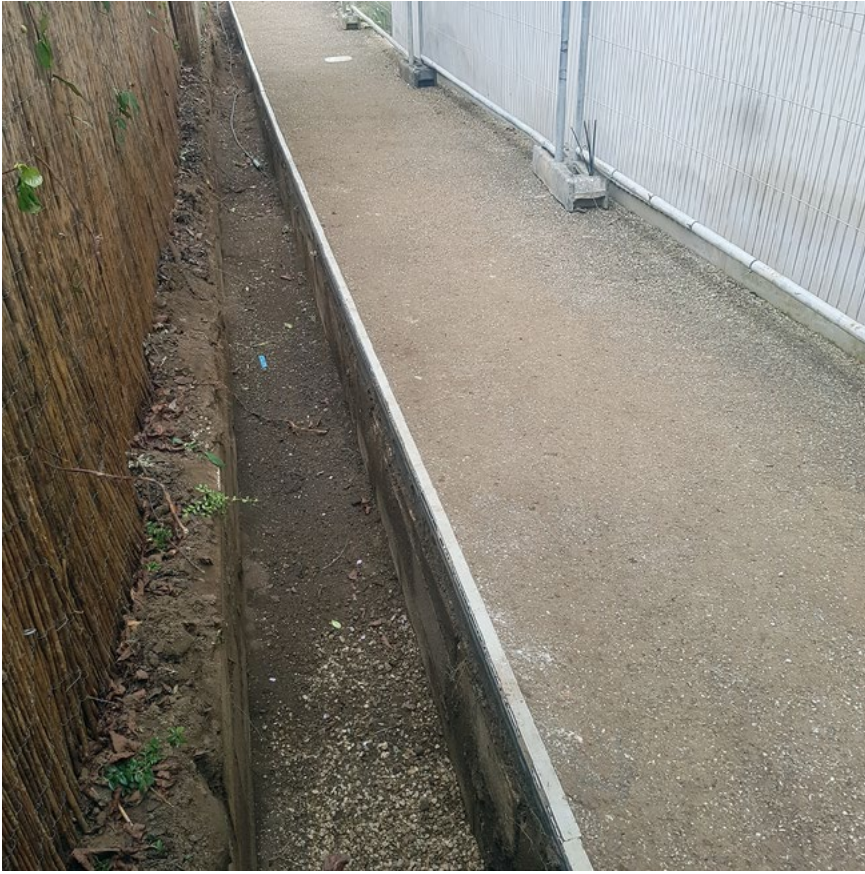
Plate 5: Trench to north of Music Rooms through modern backfill
