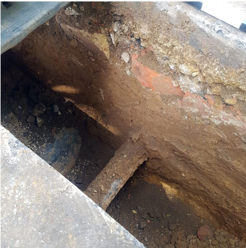
Plate 2: Services in eastern end of Trench across Mansfield Road
