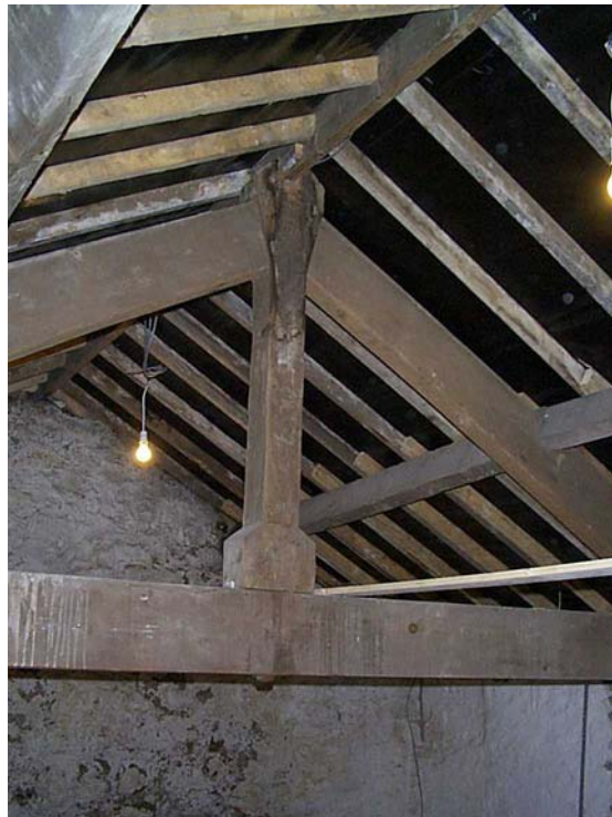
Plate 6 Kingpost truss within the farmhouse
