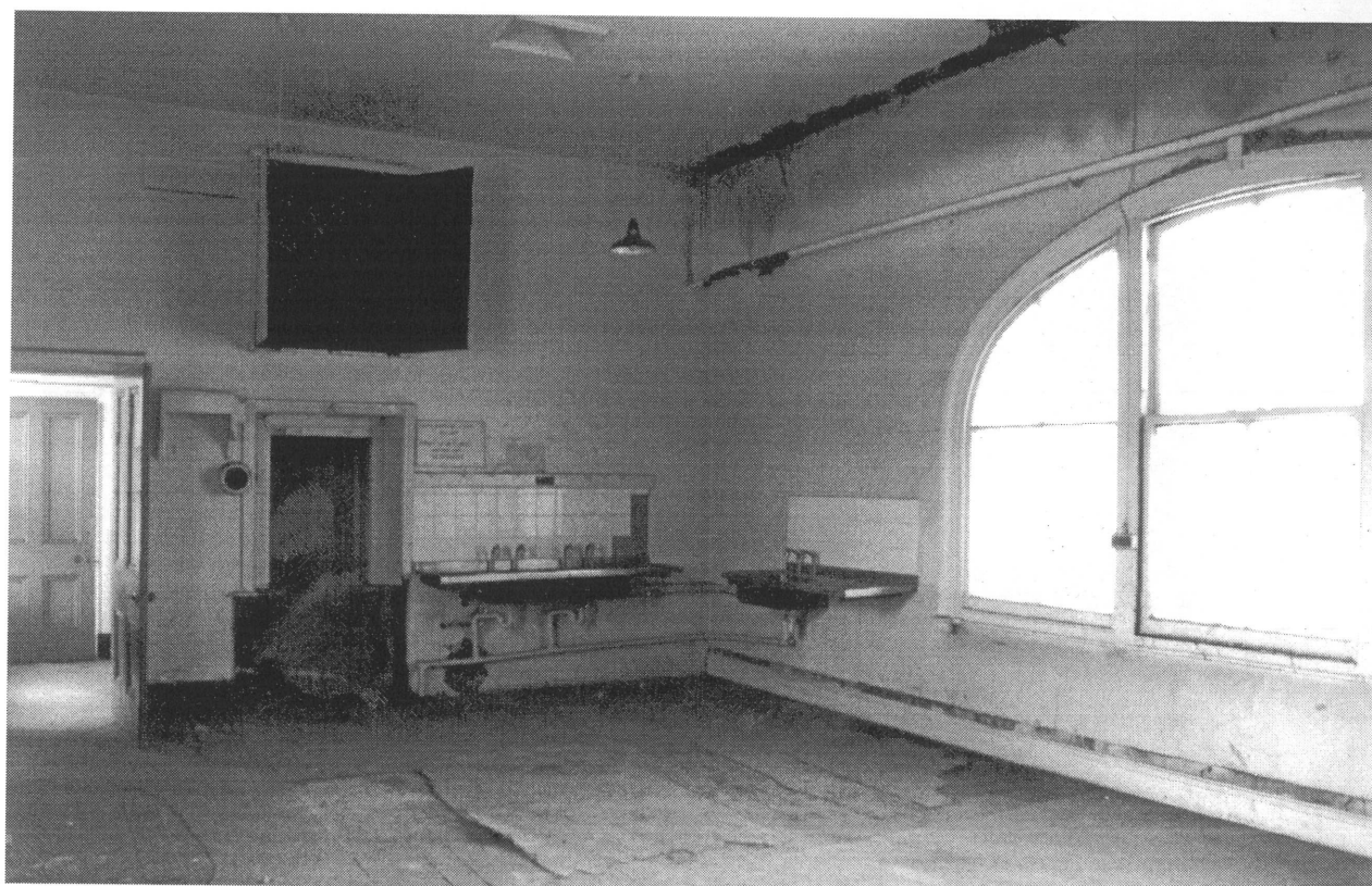
Plate 10: Room 1, First Floor, Building 6: Dumb-Waiter in situ
