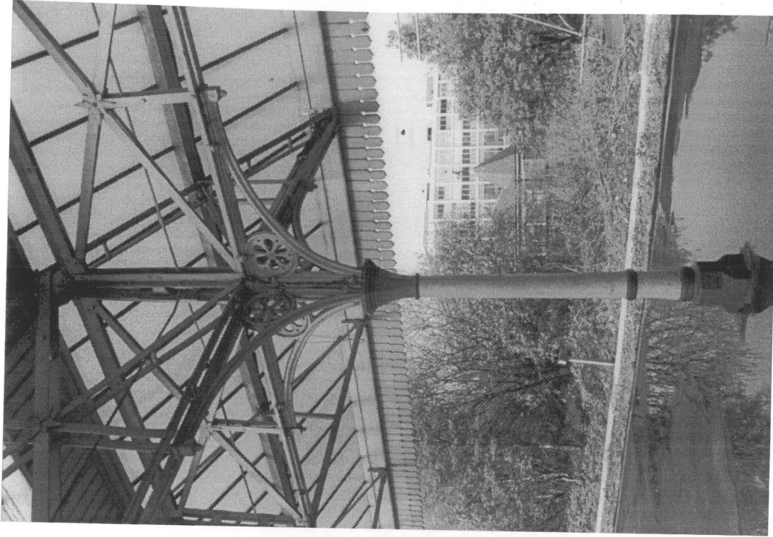
Plate 12 Column support for low-level canopy
