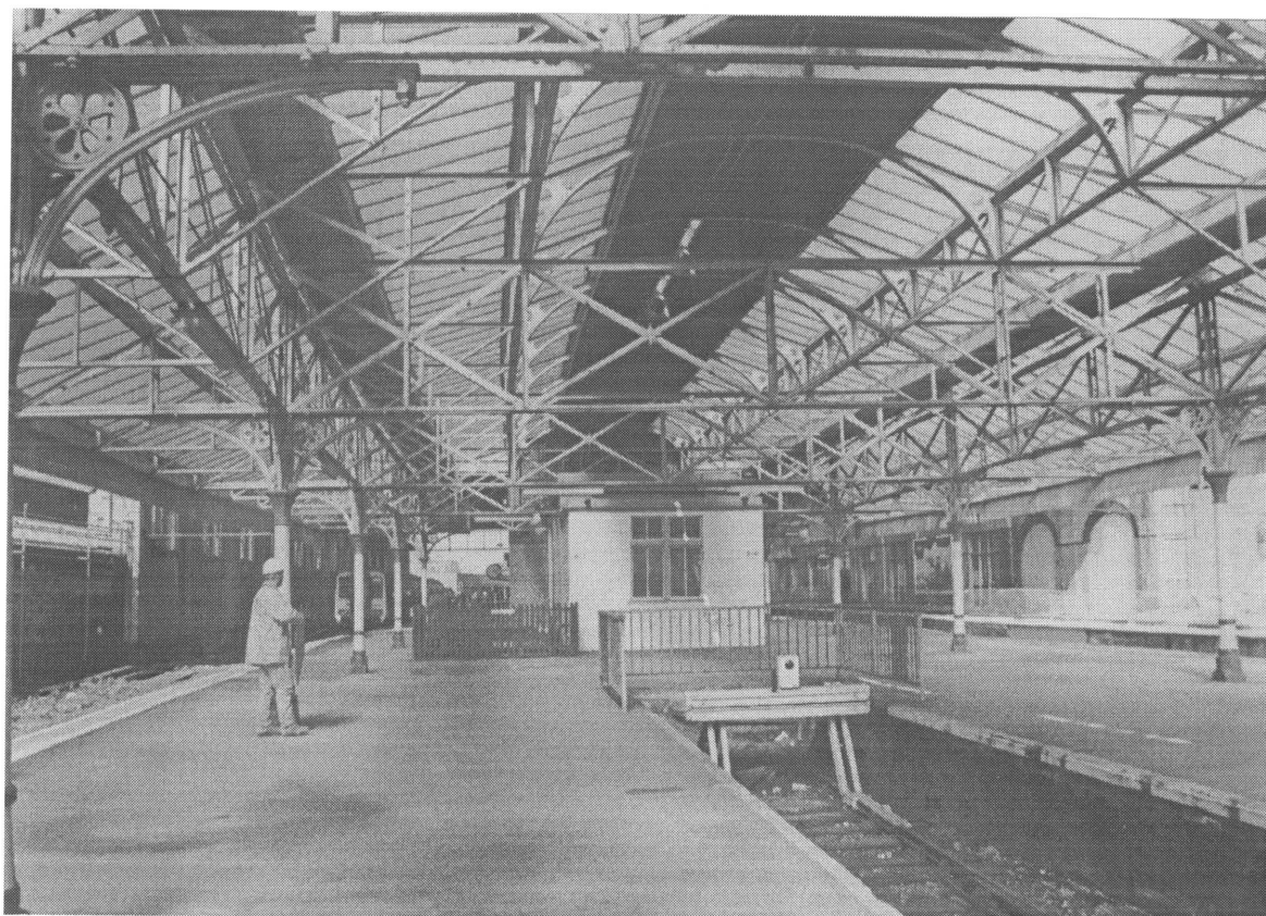
Plate 2: South end of Platform 1, showing detail of the low level canopy truss > NE
