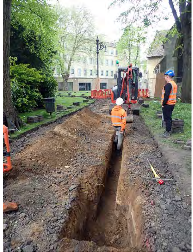
Plate 2: Cable trench excavation to east of the Minster, looking south
