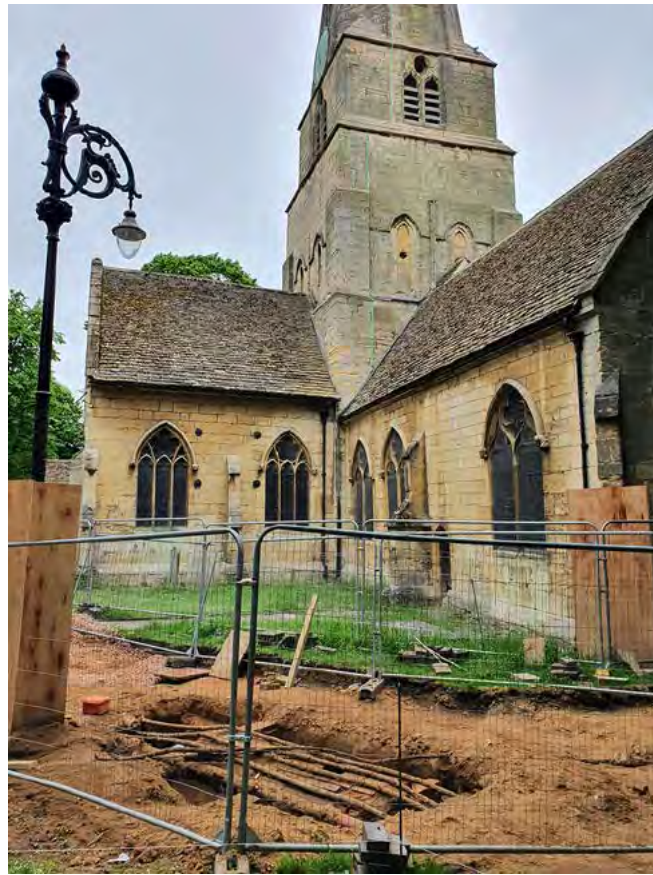
Plate 4: General view of vault 1, revealed to the south-east of the Minster
