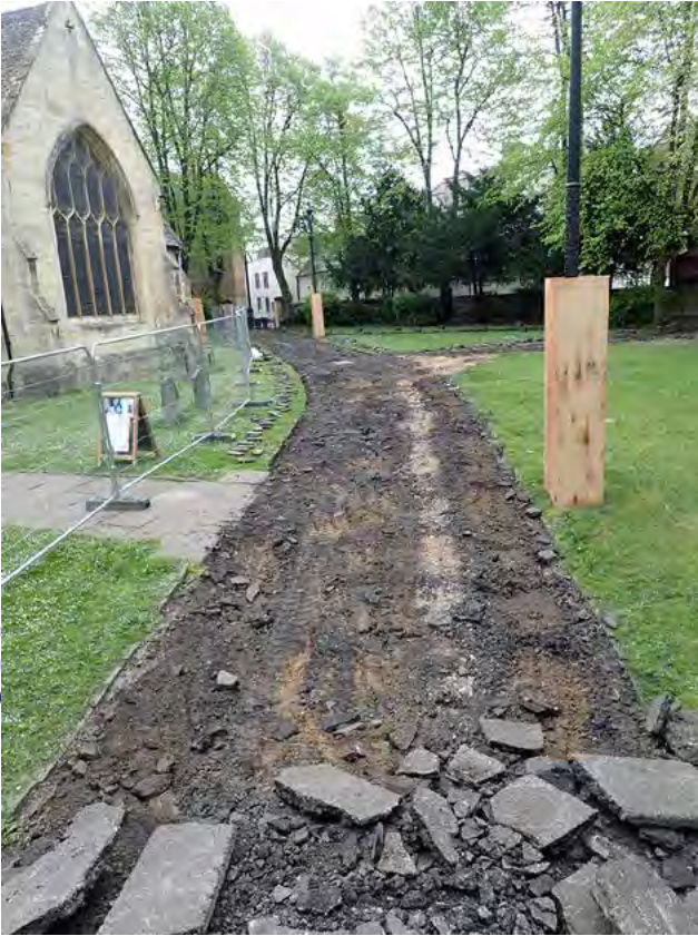
Plate 1: Pathway removal to the south of the Minster, looking east
