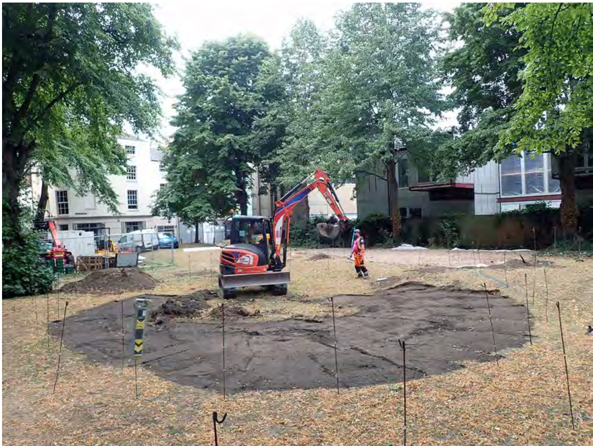
Plate 3: Topsoil stripping for seating area west of the Minster, looking south-west
