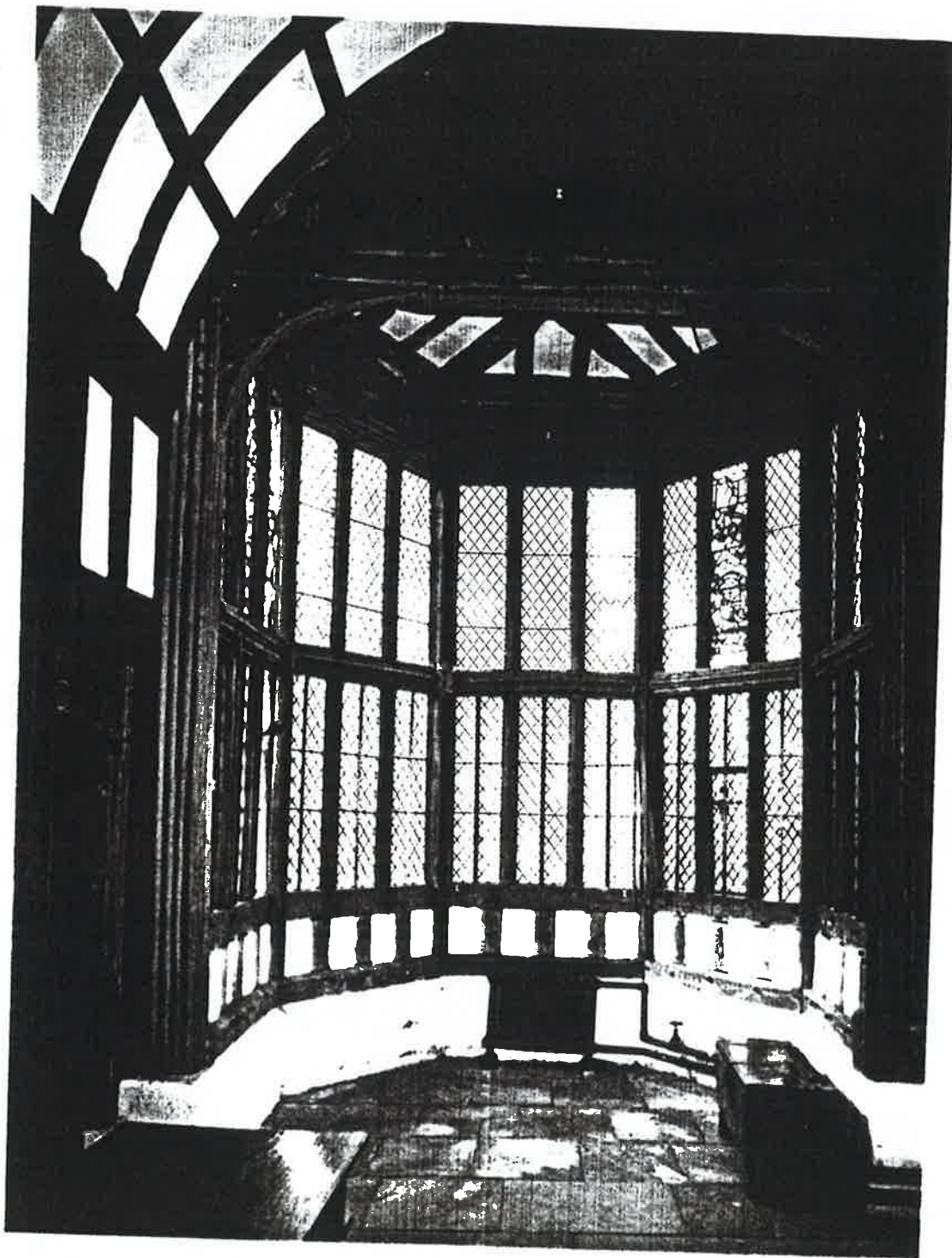
Plate 3. Internal entrance to the bay window, showing truncated post.
