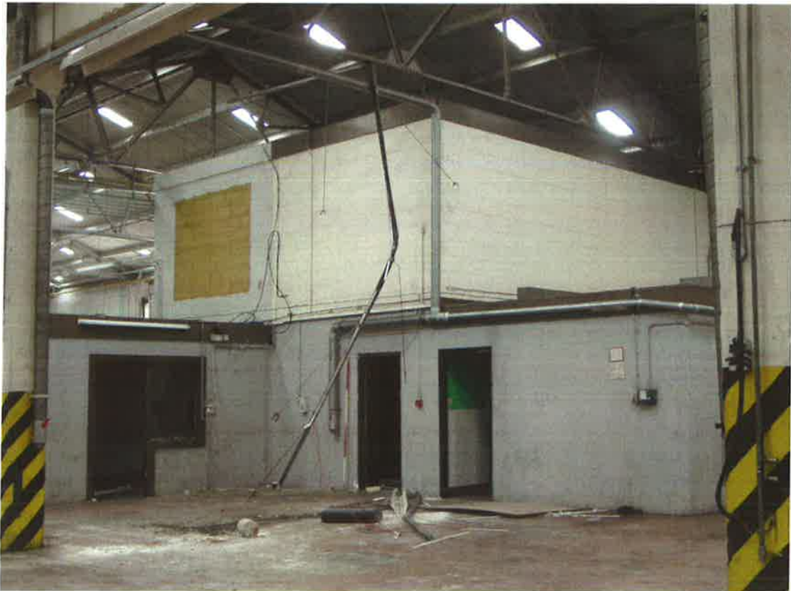
Plate 10: Later internal office buildings within the Transit Shed
