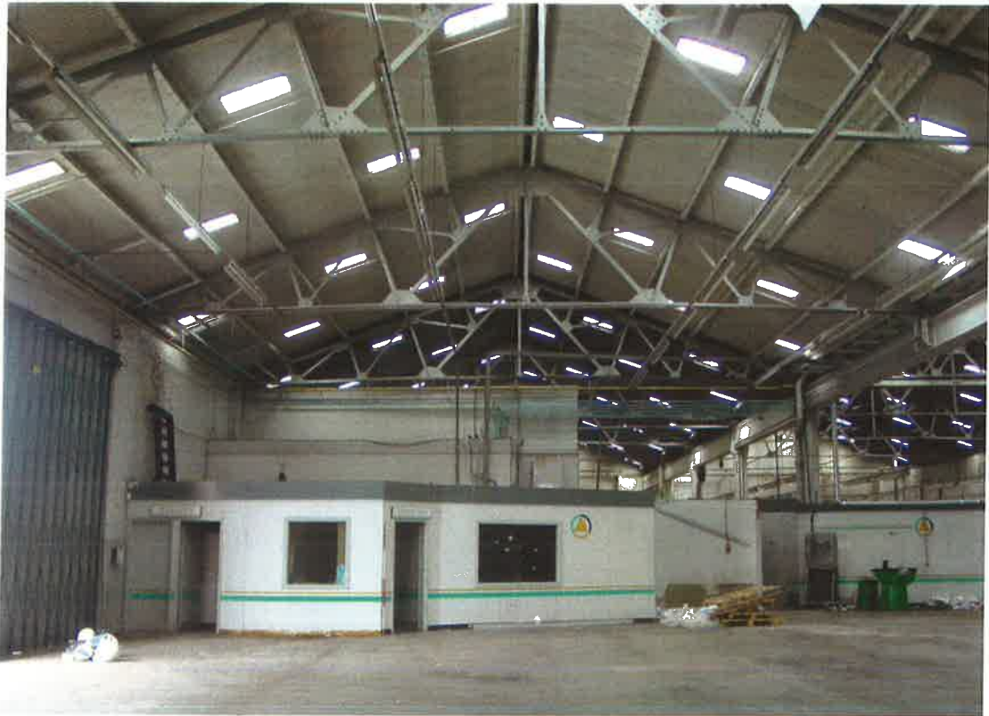
Plate 7: Central bay of the Transit Shed looking north
