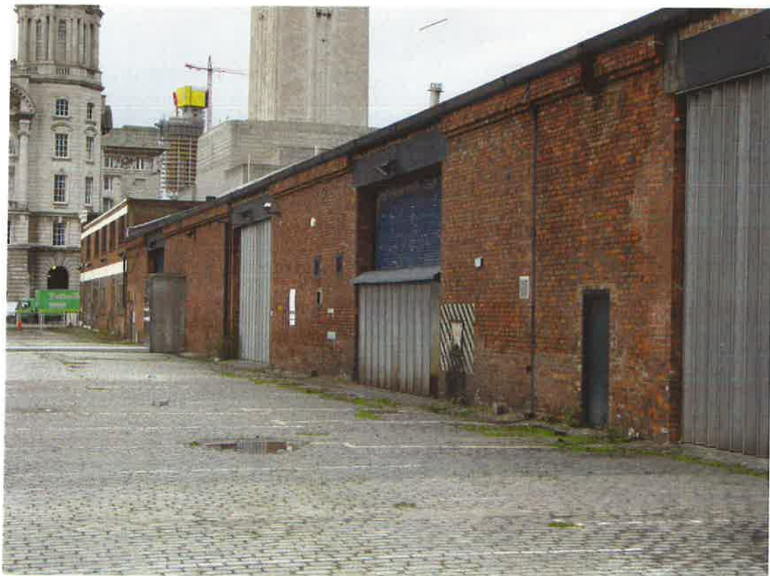
Plate 2: Western elevation (northern part) of the Transit Shed and Voss Garage
