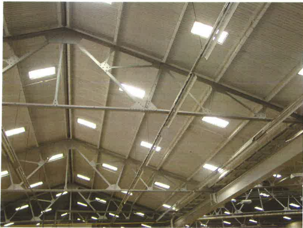
Plate 8: Truss detail of the Transit Shed roof
