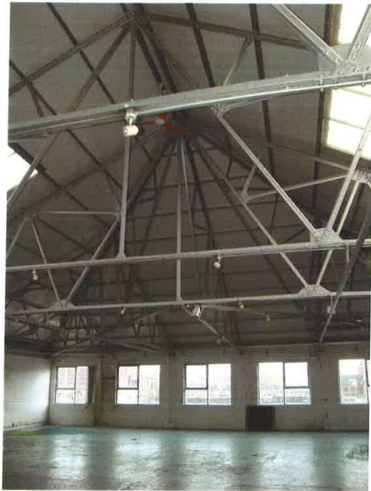
Plate 11: Steel roof structure in the Voss Garage
