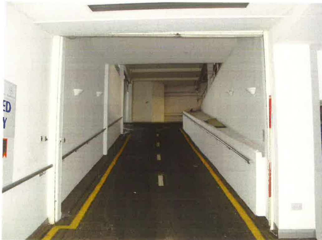
Plate 12: Car ramp inside the Voss Garage leading to the first floor
