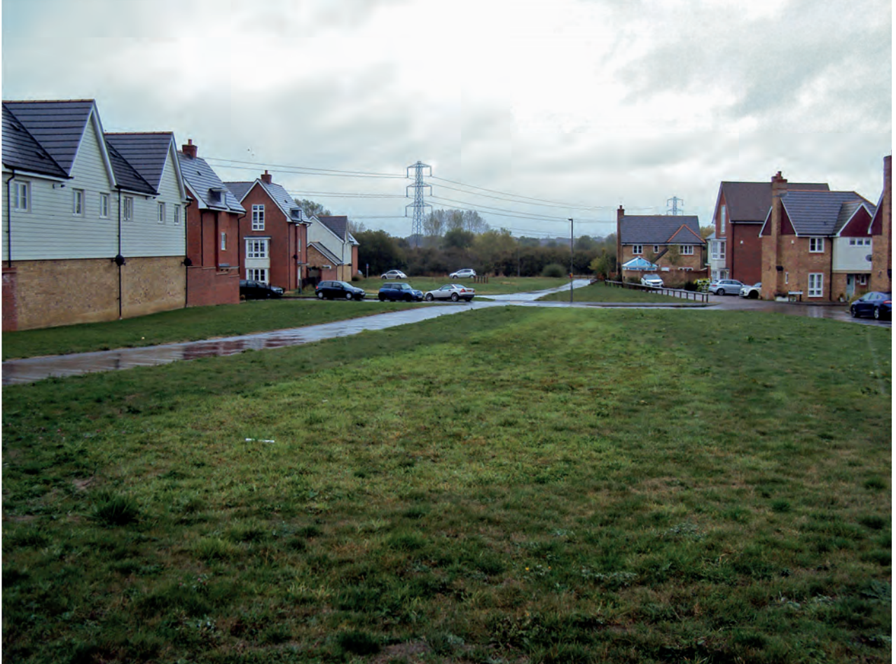
Fig. 6.5 The line of Akeman Street preserved as an open space within the Berryfields development, looking south-east towards the River Thames
