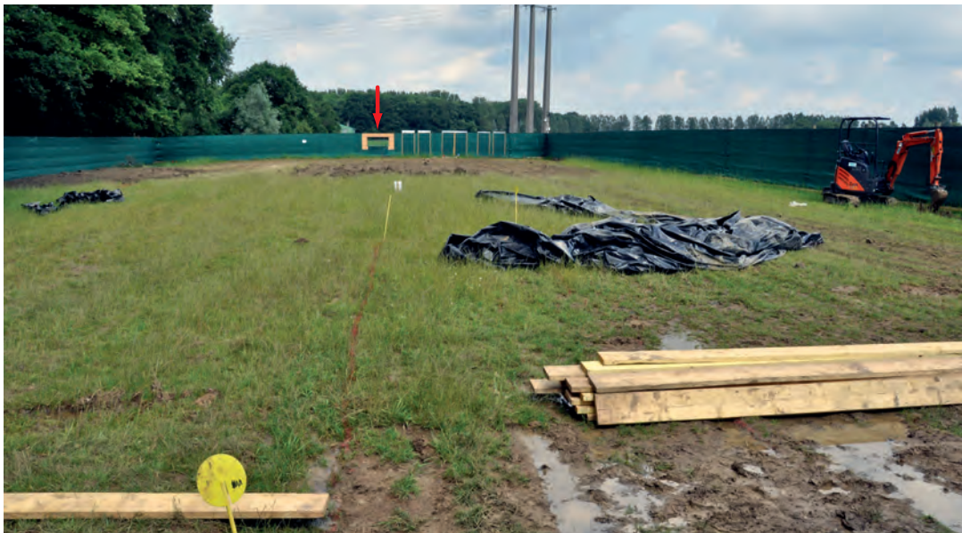
Fig. 2.4 Perimeter fence around excavation with viewing window for the public (arrowed)
