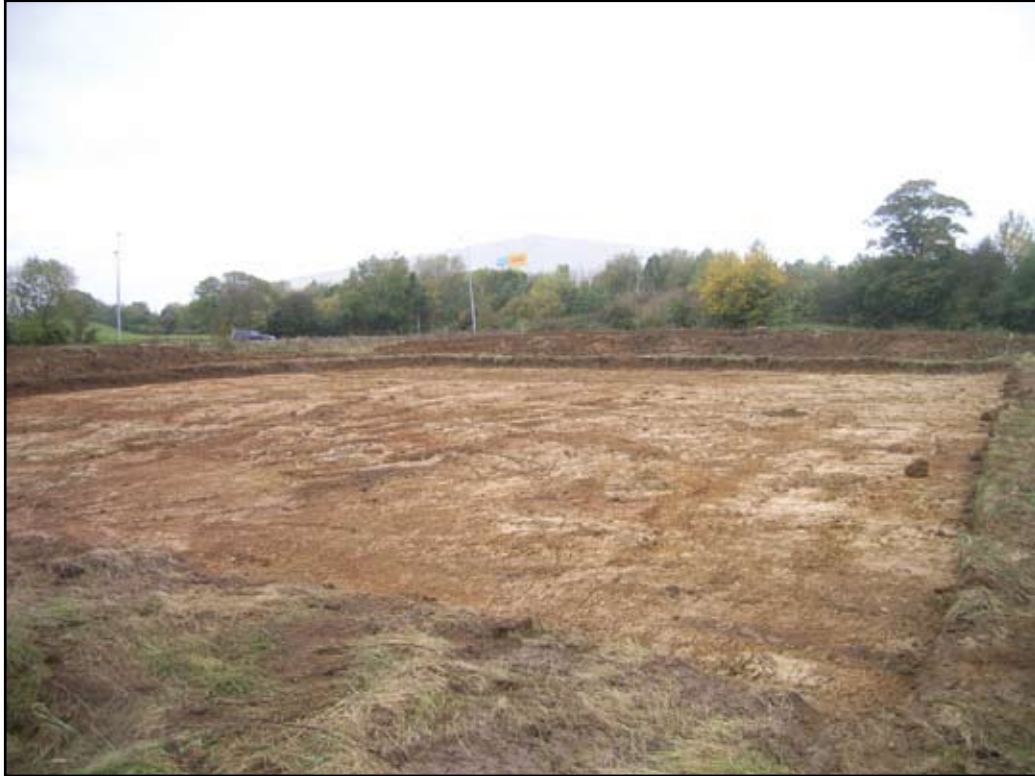
Plate 1: Excavation area, view to south
