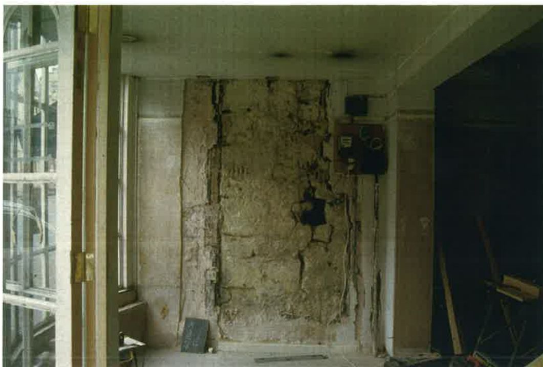
overall view of west wall of No. 41
