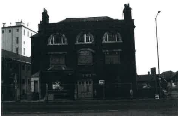
Plate 5: North elevation of 45 The Vineyard
