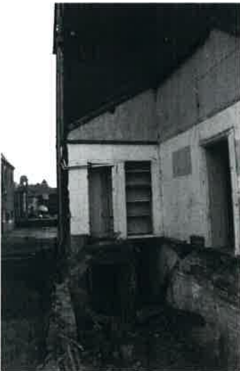
Plate 11: North-east corner of the building
