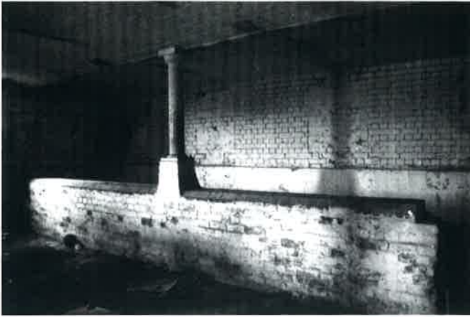
Plate 43: Steep in basement of malthouse
