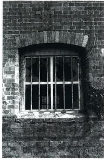
Plate 38: West elevation window detail
