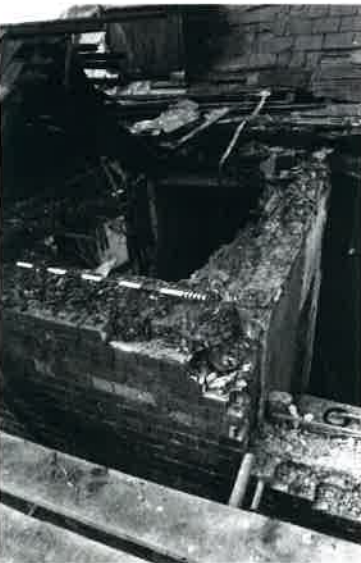
Plate 35: 2/7.0 after removal of roof
