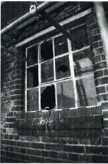
Plate 39: East elevation cast iron window detail
