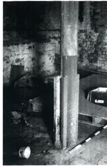
Plate 44: Detail of column in basement with bracket for removable barrier
