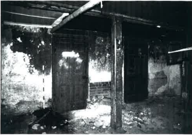
Plate 13: Cellar, B/1.0 from North-west corner
