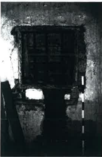
Plate 15: Internal window between B/1.2 and B/1.2
