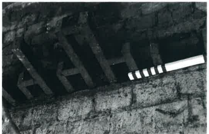
Plate 36: Grate detail in malthouse
