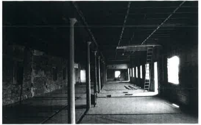
Plate 46: First floor of malthouse
