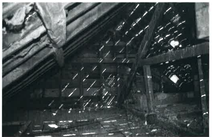
Plate 30: Queen post truss in roof
