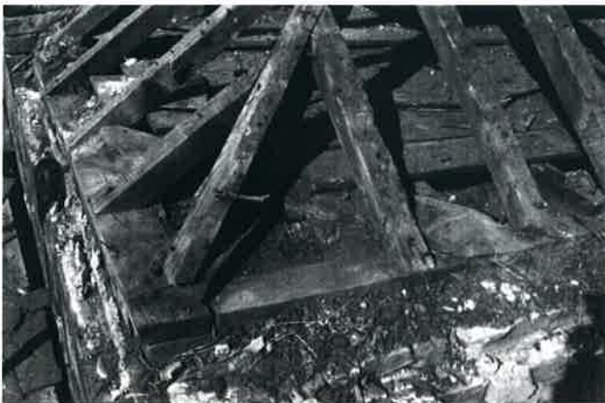
Plate 29: Corner detail of hipped roof
