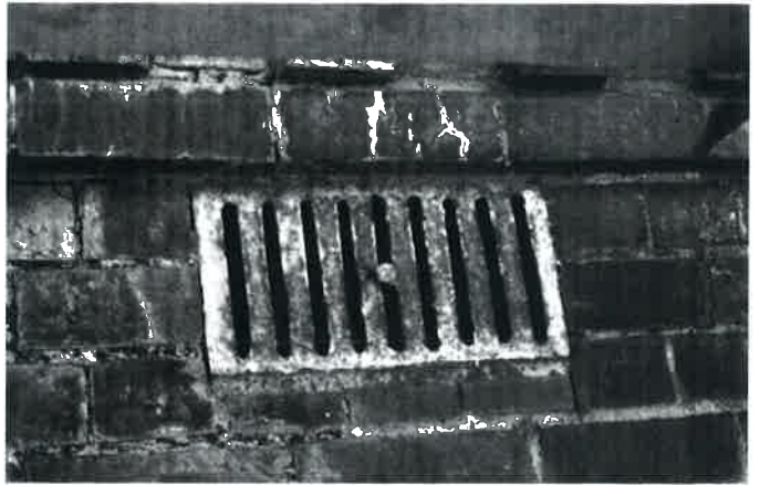
Plate 40: Malthouse vent cover detail
