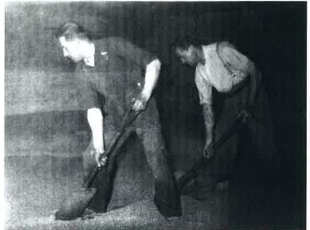
Plate 2: Typical historical view of maltings workers turning the malt in kiln
