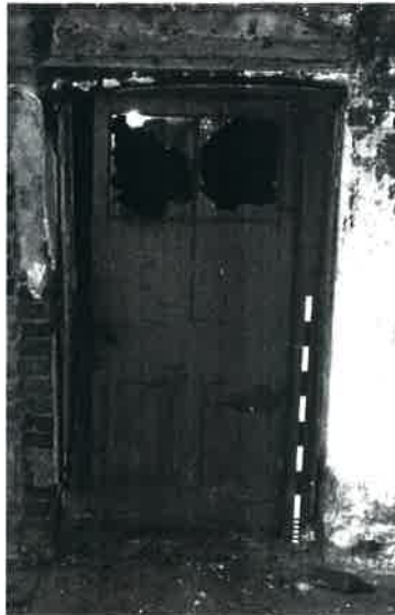
Plate 24: Central door in North wall of B/6.0
