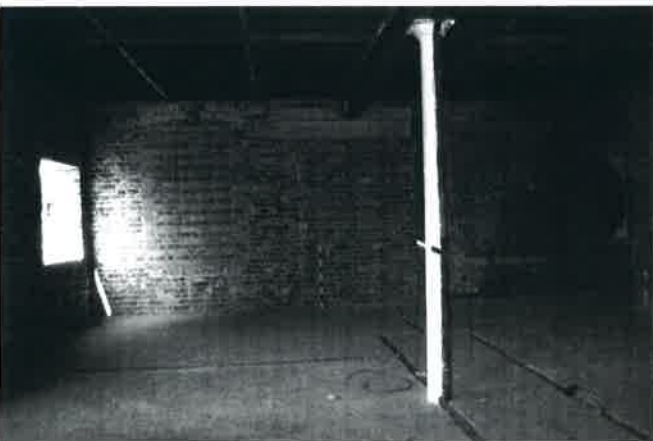
Plate 47: First floor of malthouse
