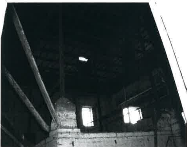
Plate 53b: View up towards drying floor above kiln
