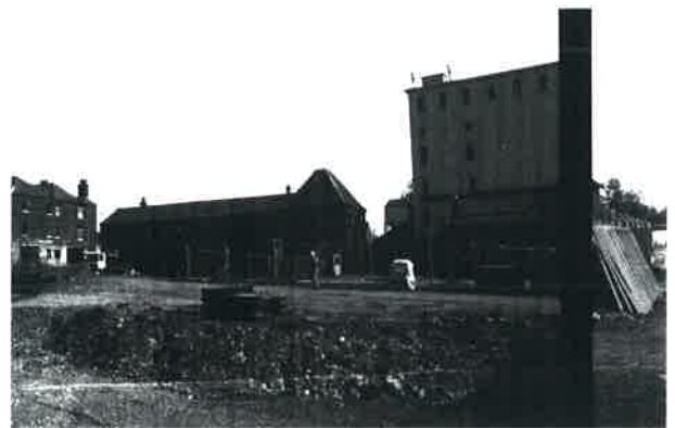
Plate 4: General view from the South-west
