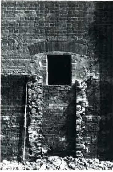
Plate 37: Blocked door in Bay 1 of West elevation of malthouse
