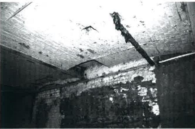
Plate 45: Brick-vaulted ceiling in basement of malthouse, note hatch
