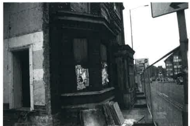
Plate 6: Bay window in North elevation of 45 The Vineyard
