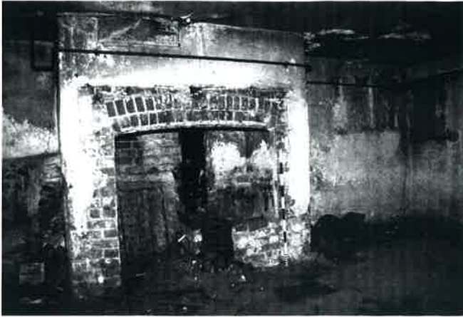
Plate 19: Fireplace in B/3.0
