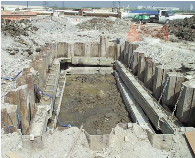
Plate 22 Cofferdam excavation 3880TT, Swanscombe
