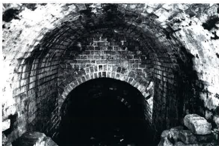
Plate 3: Interior of ice house from upper chamber
