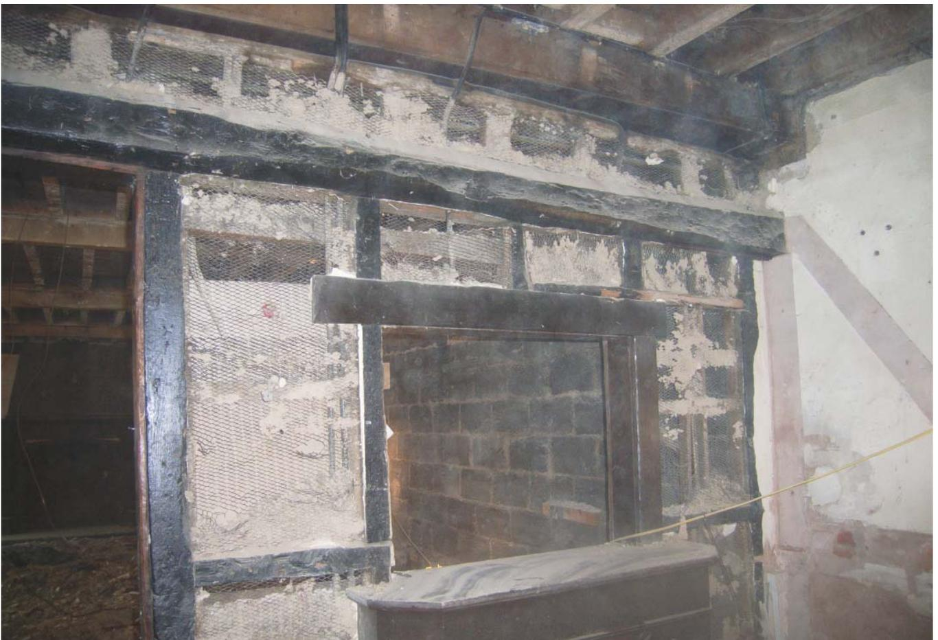
Plate 12: North side of historic frame after partial clearance of 20th-century plaster
