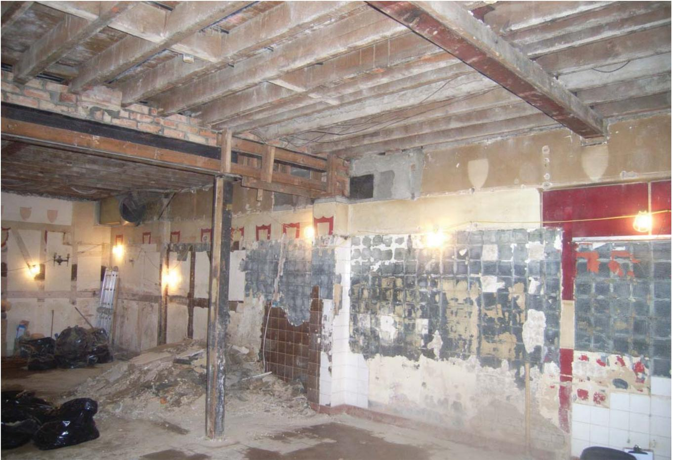
Plate 19: Area 4 and 5 after removal of partition
