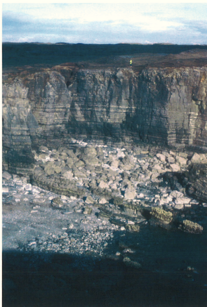
View of the eroded sections, to the east.
