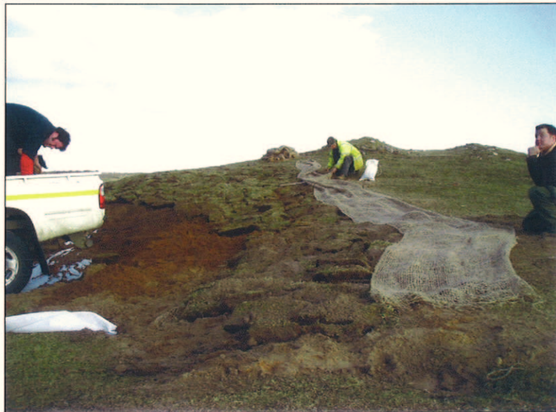
Repairs in progress - view to the east
