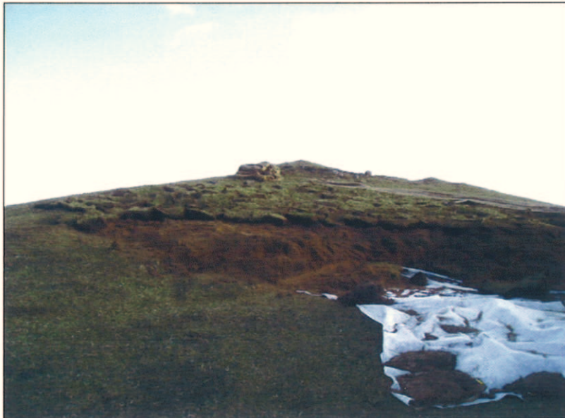
Repairs in progress - view to southeast
