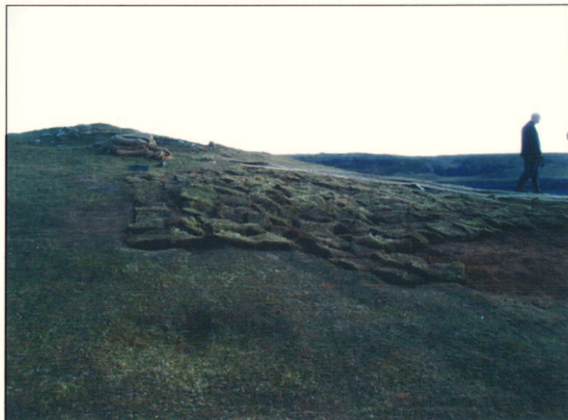
Repair completed - view to south
