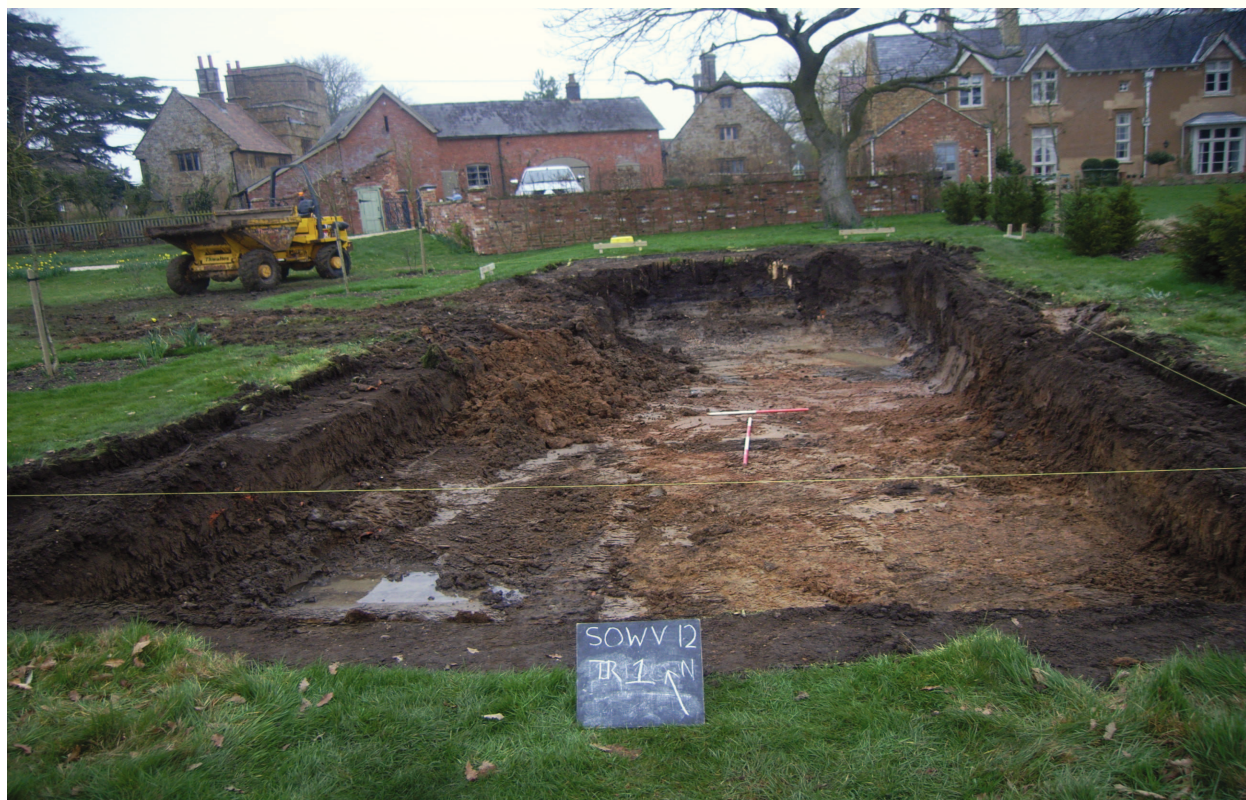
Plate 4: Swimming pool footprint excavated to natural geology
